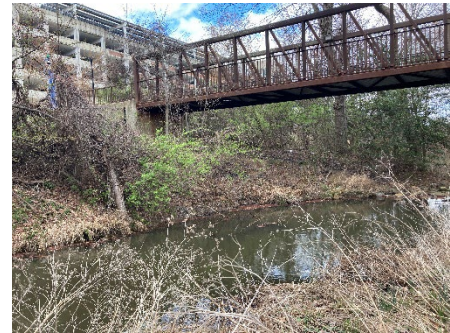
Figure 14: Pedestrian bridge from Terrapin Trail Parking Garage (Photo by the author)
