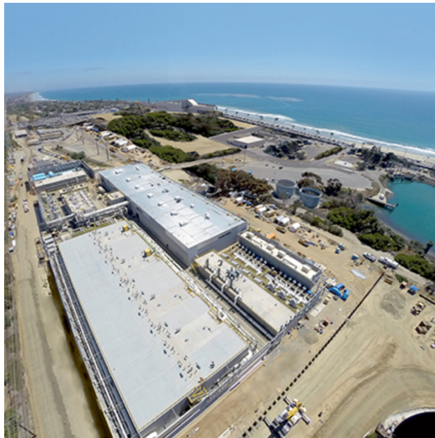
Aerial view of the Carlsbad Seawater Desalination Plant
