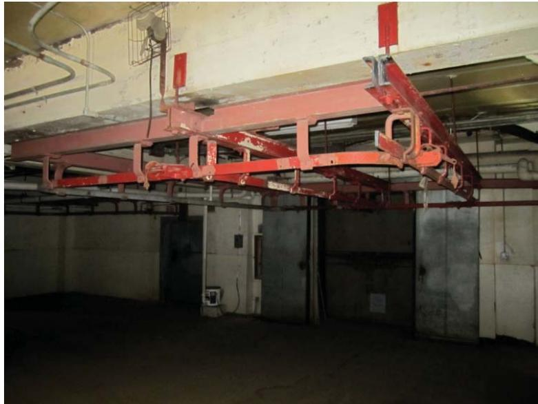
**Figure A11: View of suspended meat rails hanging from the ceiling**
