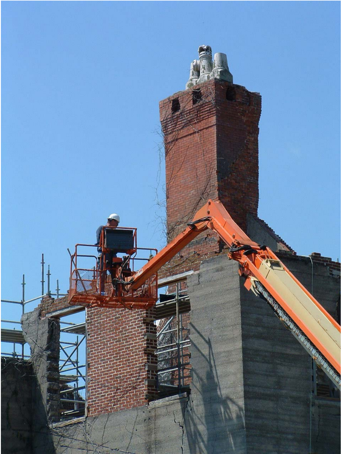
Figure 20. Brick and mortar conservation treatment at Dungeness Mansion ruins, Cumberland Island, Georgia (Photo by J. Ruck, March 2008).
