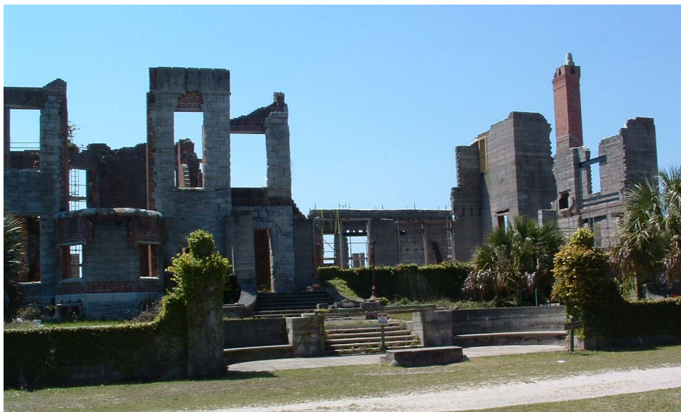
Figure 16. Dungeness Mansion ruins, Cumberland Island, Georgia (Photo by J. Ruck, March 2008).
