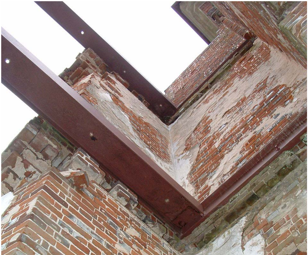
Figure 22. Steel structural reinforcement utilized for stabilization of Rosewell ruins in Gloucester, Virginia (Photo by J. Ruck, April 2008).
