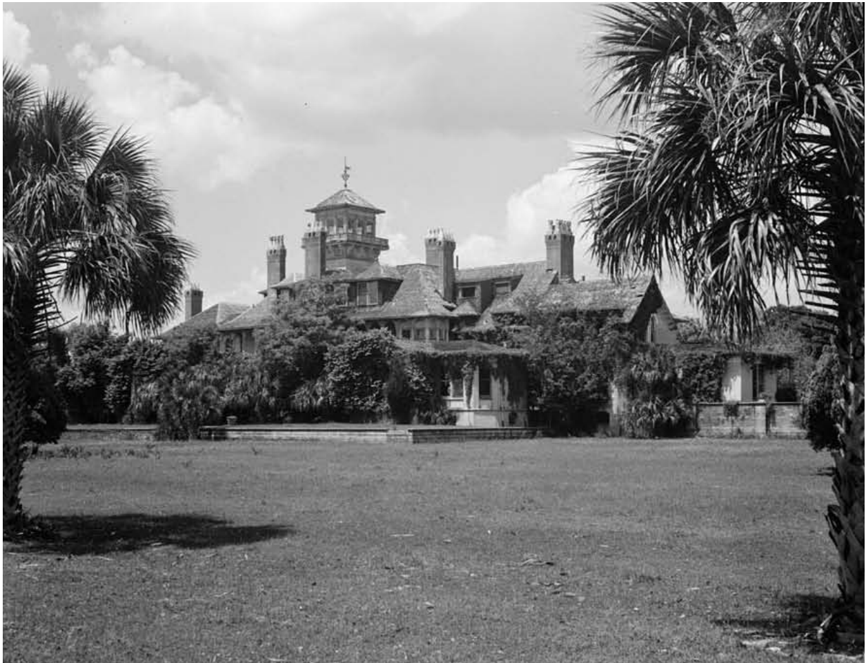
Figure 19. Front and north side elevations of Dungeness Mansion prior to ruination (Photo by Philip E. Gardner for the Historic American Buildings Survey, 1958; Available from the Library of Congress at http://hdl.loc.gov/loc.pnp/hhh.ga0298 ; Accessed May 2008).
