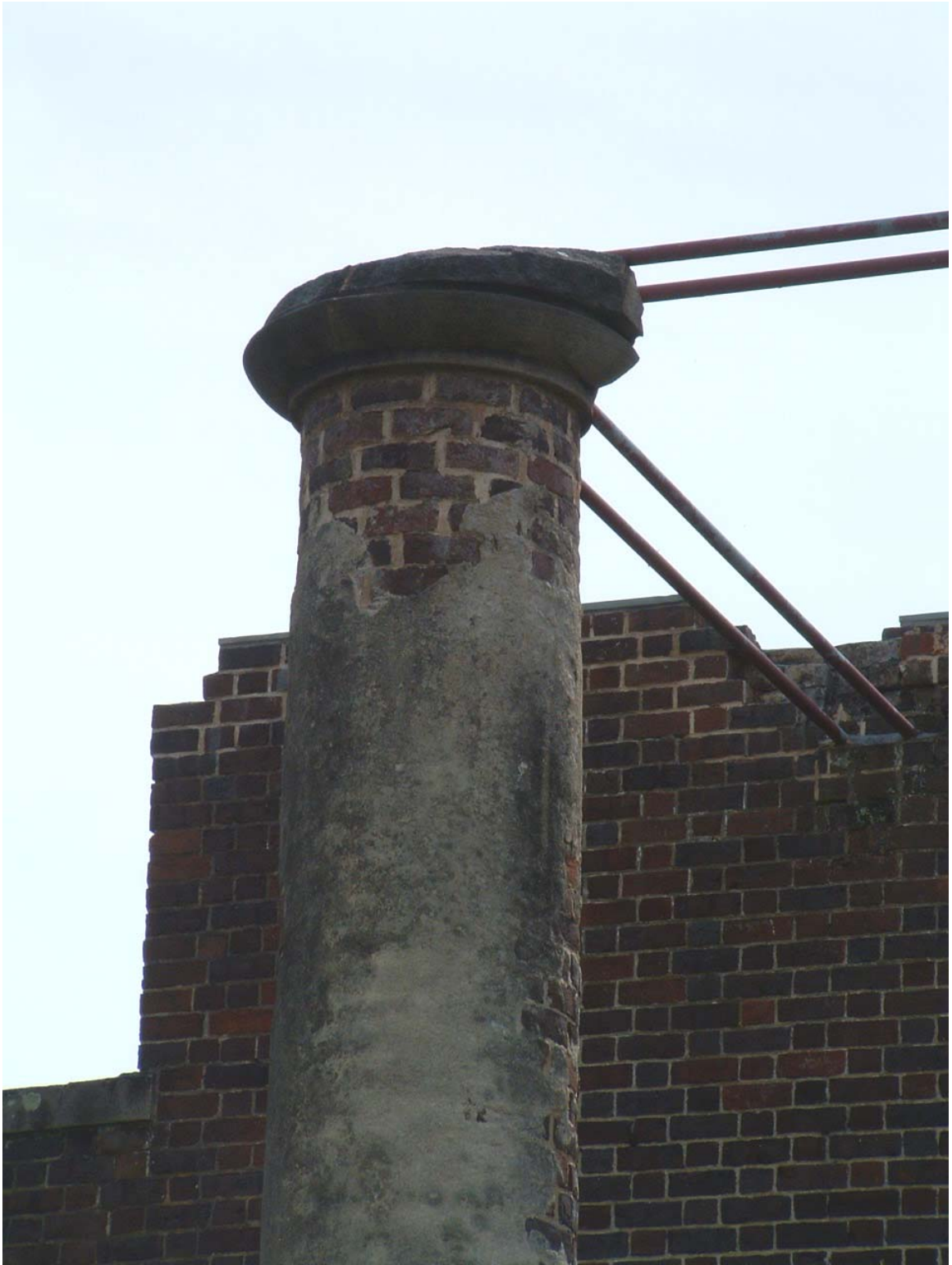
Figure 25. Column of the Old Governor's Mansion at Barboursville Vineyards, with steel reinforcement (Photo by J. Ruck, April 2008).
