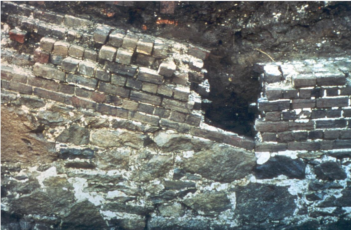
Figure 3.4 shows a portion of the west garden wall excavated by Glenn Little during the 1967 field season. The photograph shows the wall's fieldstone and mortar base sloping down toward King George Street. Atop the fieldstone, brick courses were laid to correspond with the terracing of the garden surface (Little 1967)
