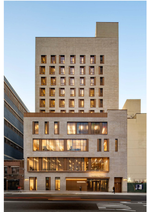
Figure 21. Exterior Image of the Building
