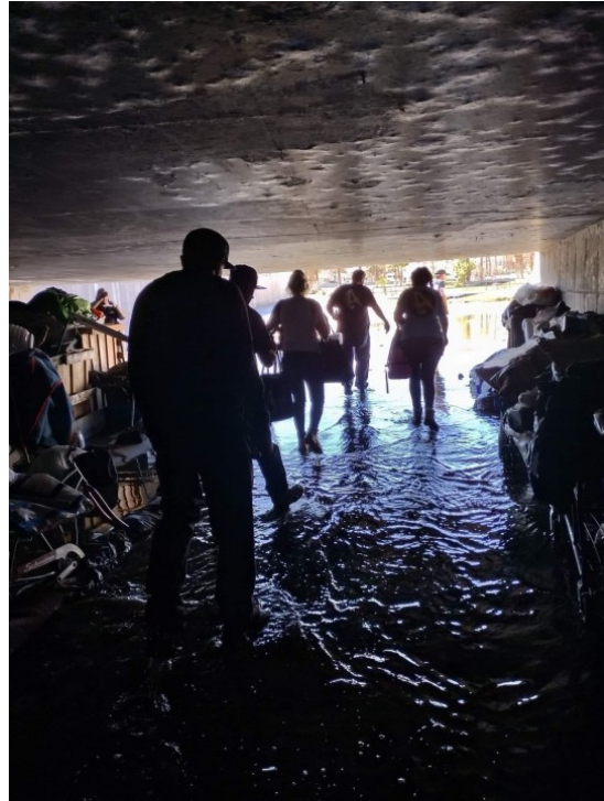
Figure 1. Flooding of the Las Vegas Tunnel Encampments
