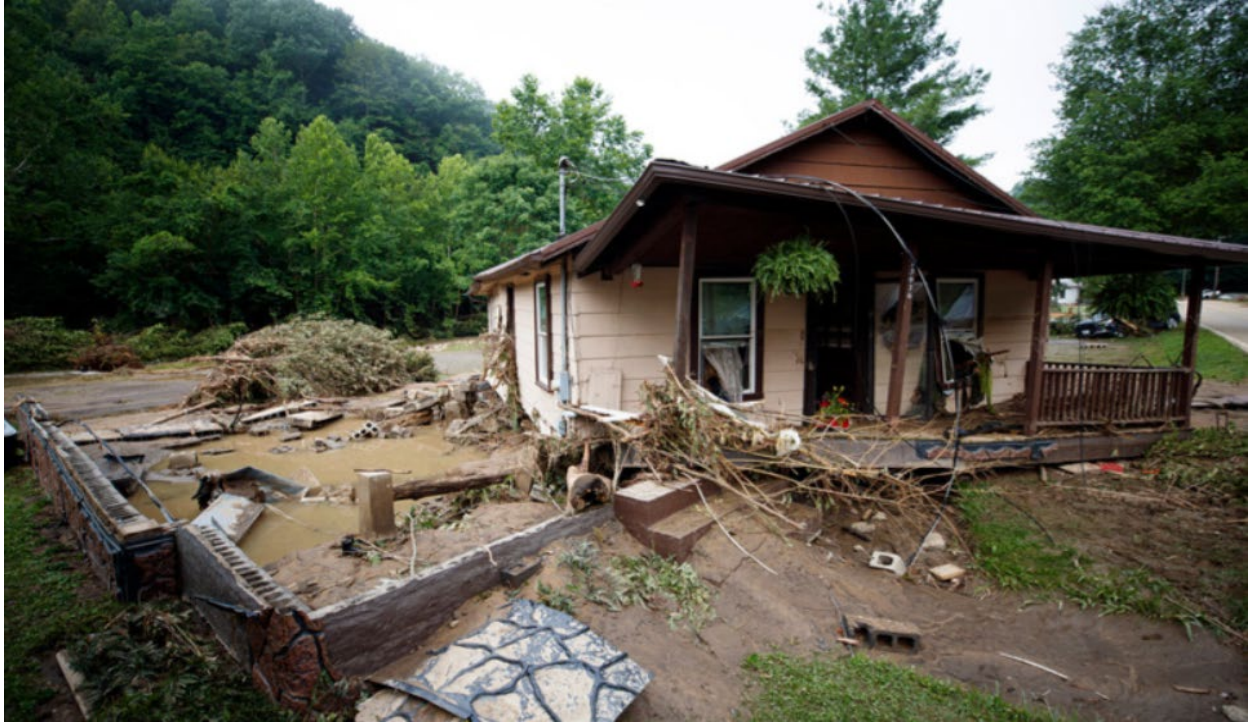
Fig. 22: house moved from its foundation in Whitewood, VA. 74
