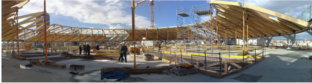
Illustration 26: View of Dome during Construction (source: Rogers Stirk Harbour + Partners)
