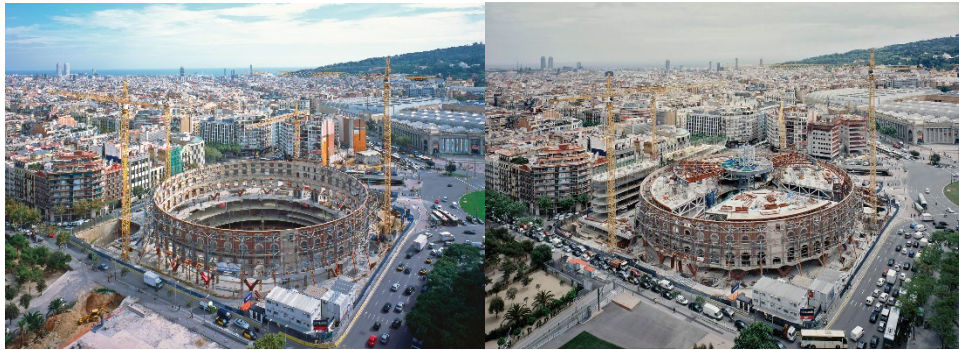
Illustration 24: Aerial View of Construction Progress Showing the Retention of the Original Façade (source: Rogers Stirk Harbour + Partners)
