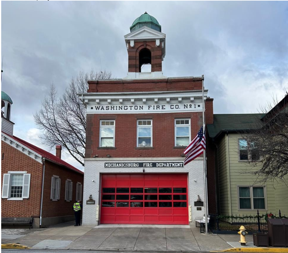
Photo 3 of 19: The Washington Fire Company building at 53 E Main Street, facing northwest.
