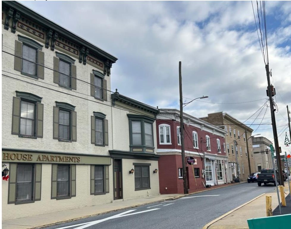
Photo 7 of 19: 20-8 N Market Street and 1-8 E Main Street, facing south.
