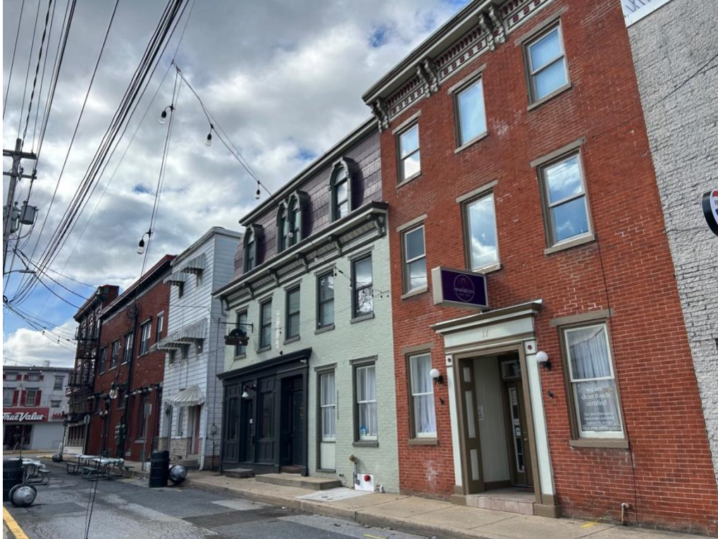
Photo 9 of 19: 7-17 N Railroad Avenue, facing south.
