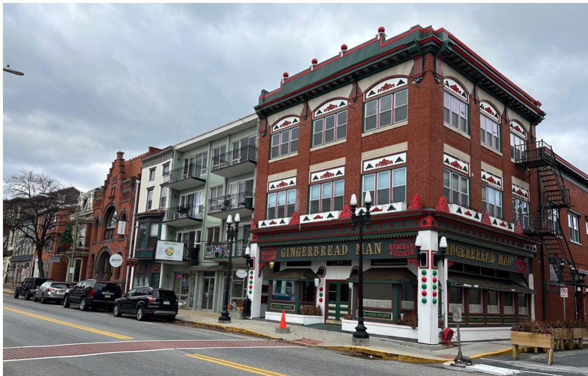
Photo 8 of 19: 26-46 W Main Street, facing northwest.
