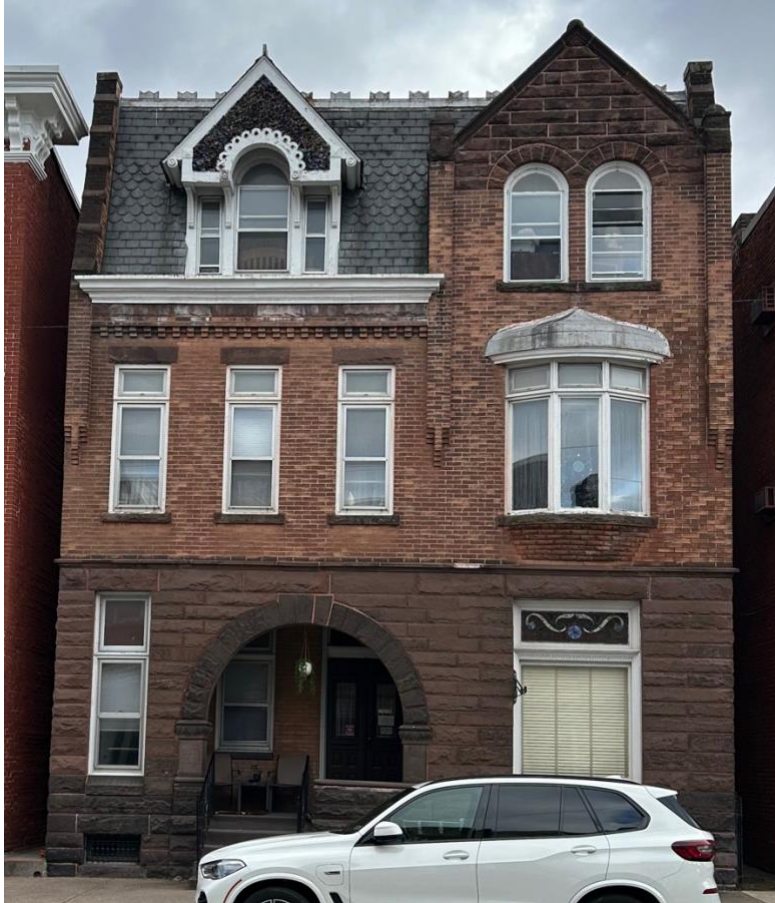
Photo 13 of 19: 55 W Main Street, facing southeast.
