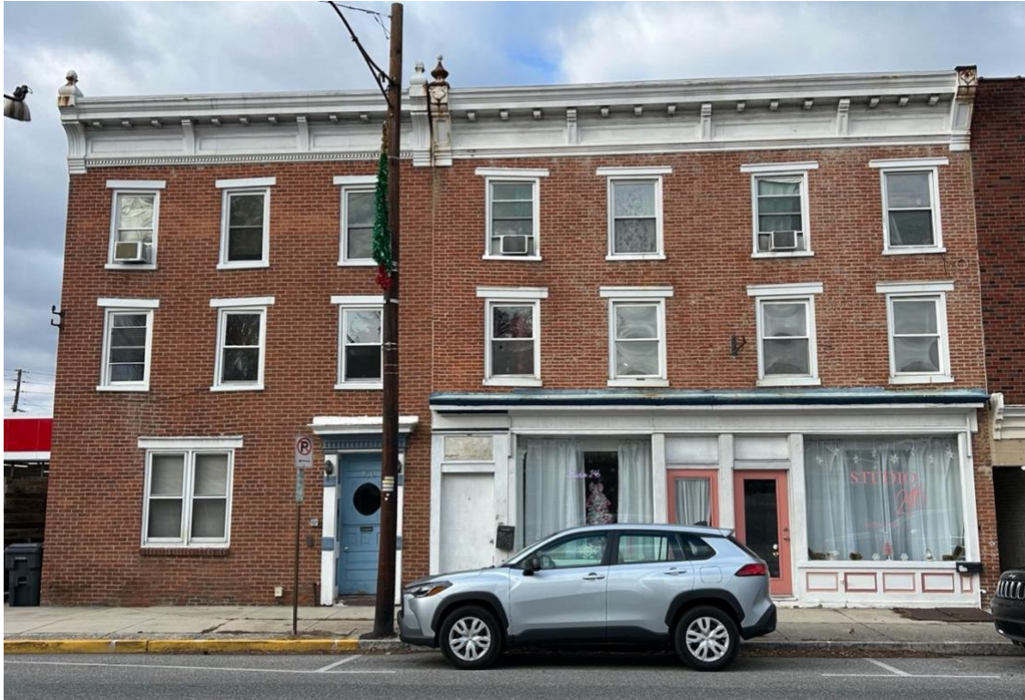
Photo 18 of 19: 130-128 W Main Street, facing northeast. Includes prior 126 W Main Street.
