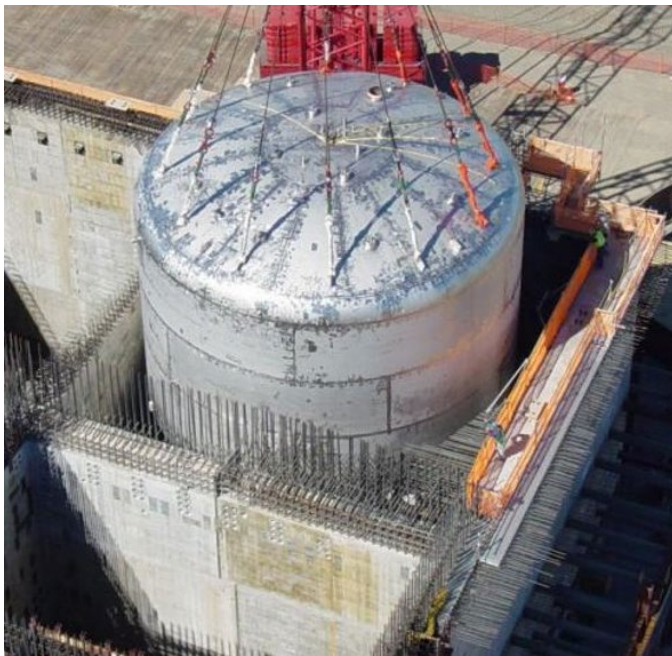
Figure 2. "Black Cell" Construction with a 38-ft-diameter Vessel with 16 PJM's. Image excerpted from [8].
