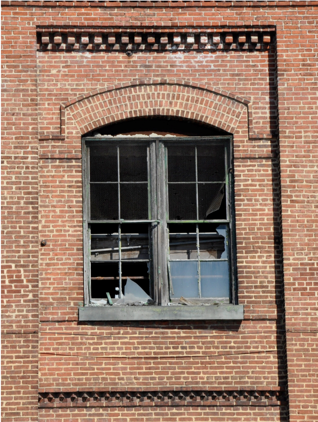
Figure 31: Detail of brick corbelling (photo by author).
