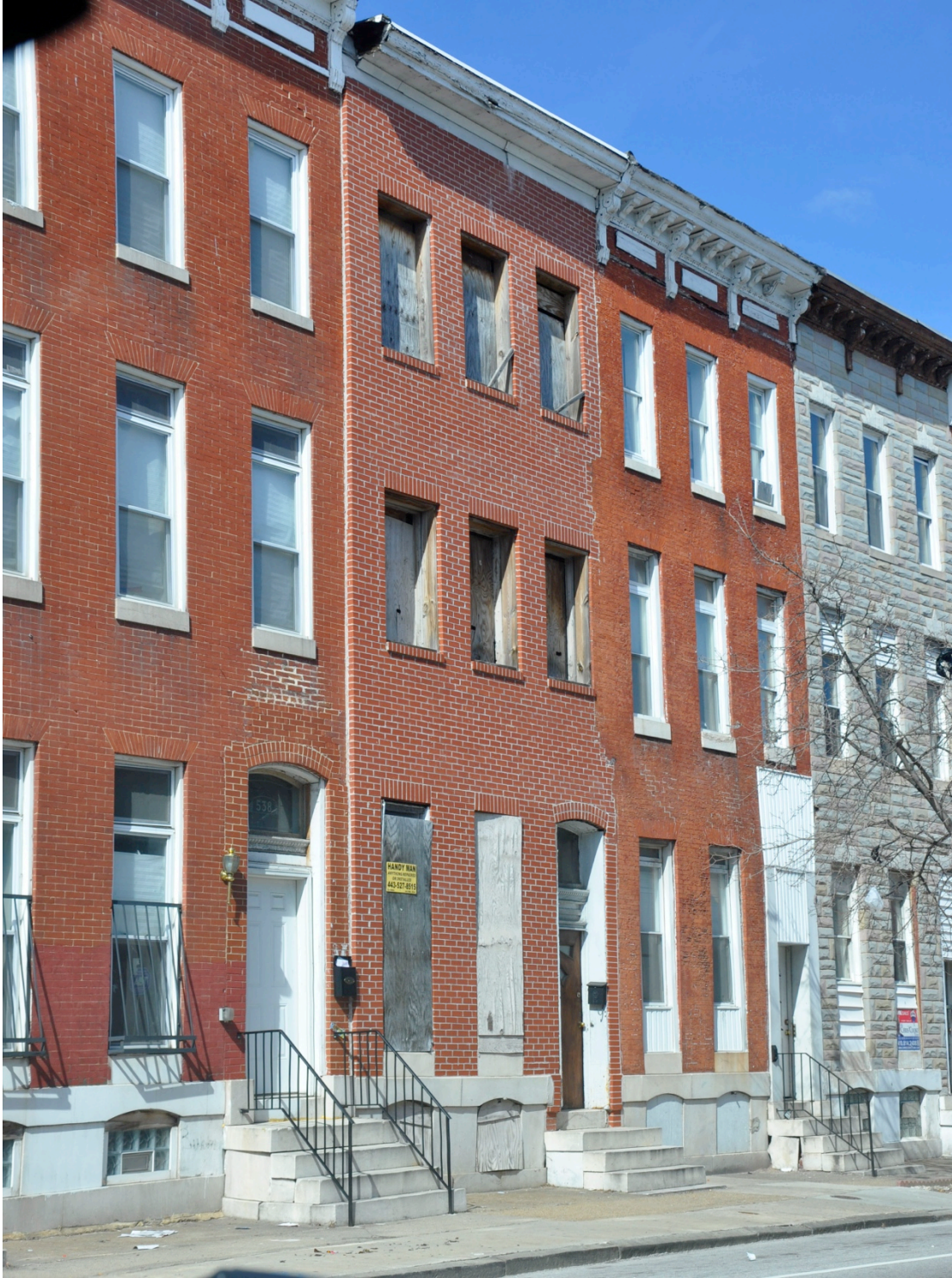
Figure 50: Example of 3 story, 3 bay Italianate style rowhouses common in the neighborhood around the Ice House (photo by author).
