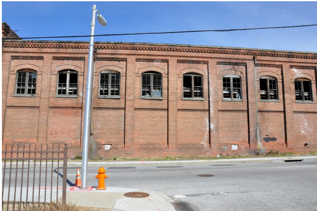
Figure 38: Detail of tank house (photo by author).
