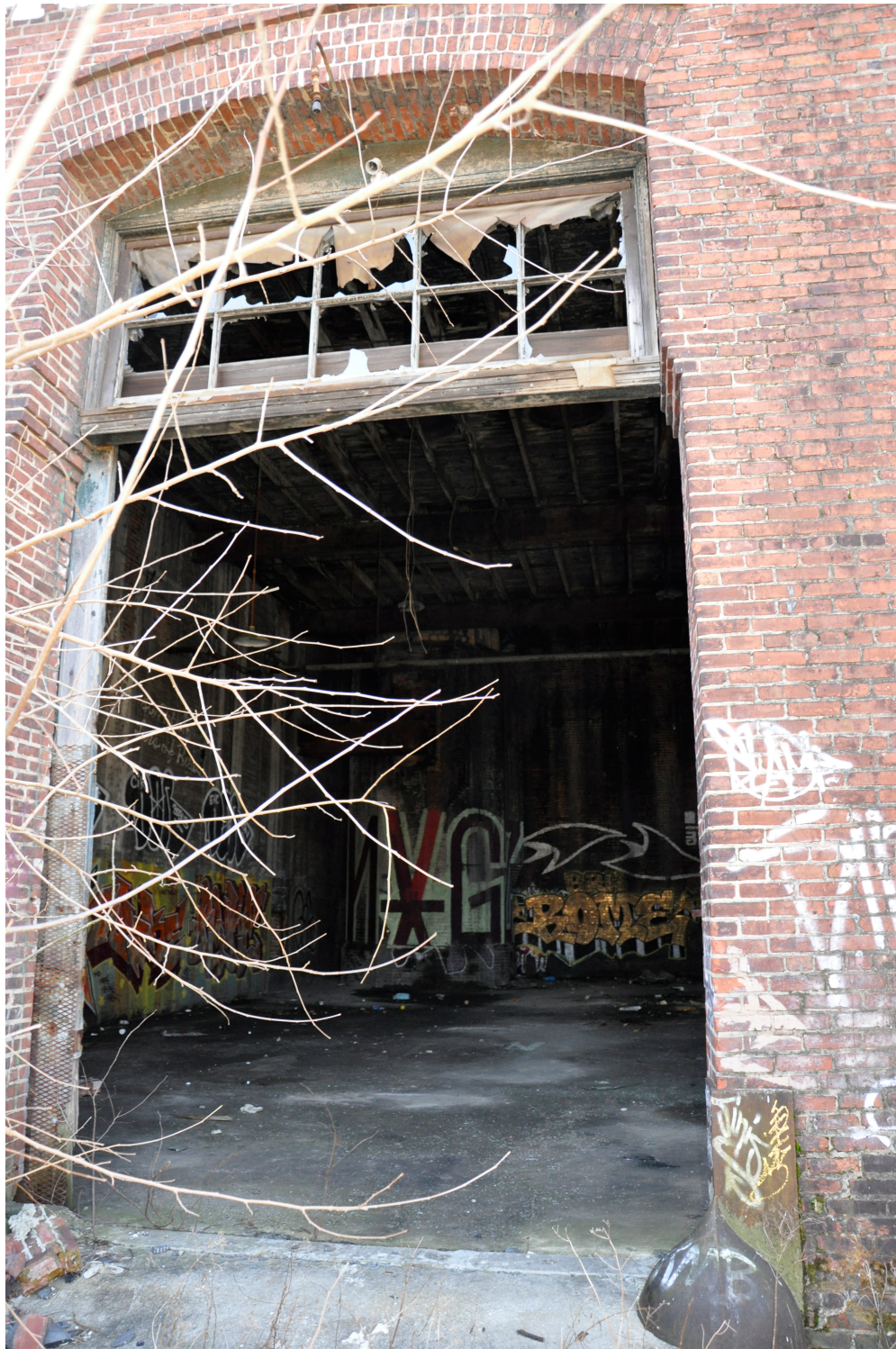
Figure 35: Service entrance to engine room (photo by author).
