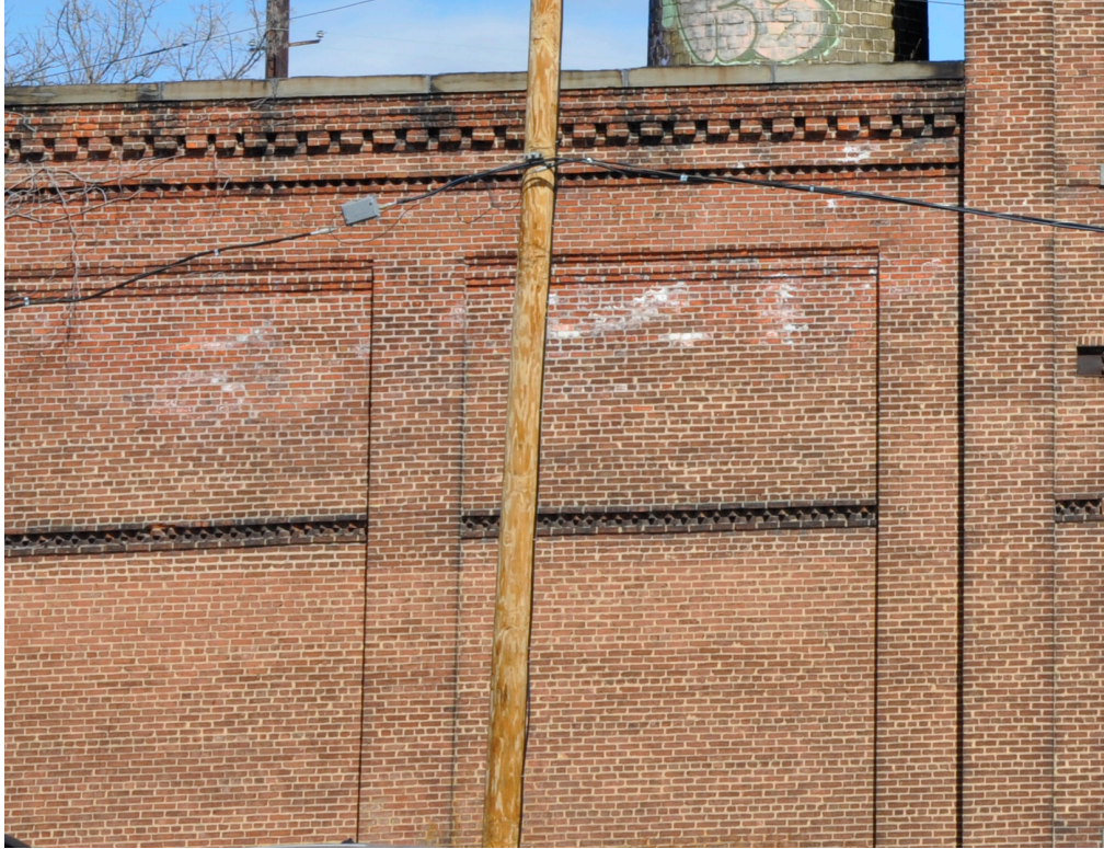
Figure 33: Detail mimicked window openings on engine room's front façade (photo by author).
