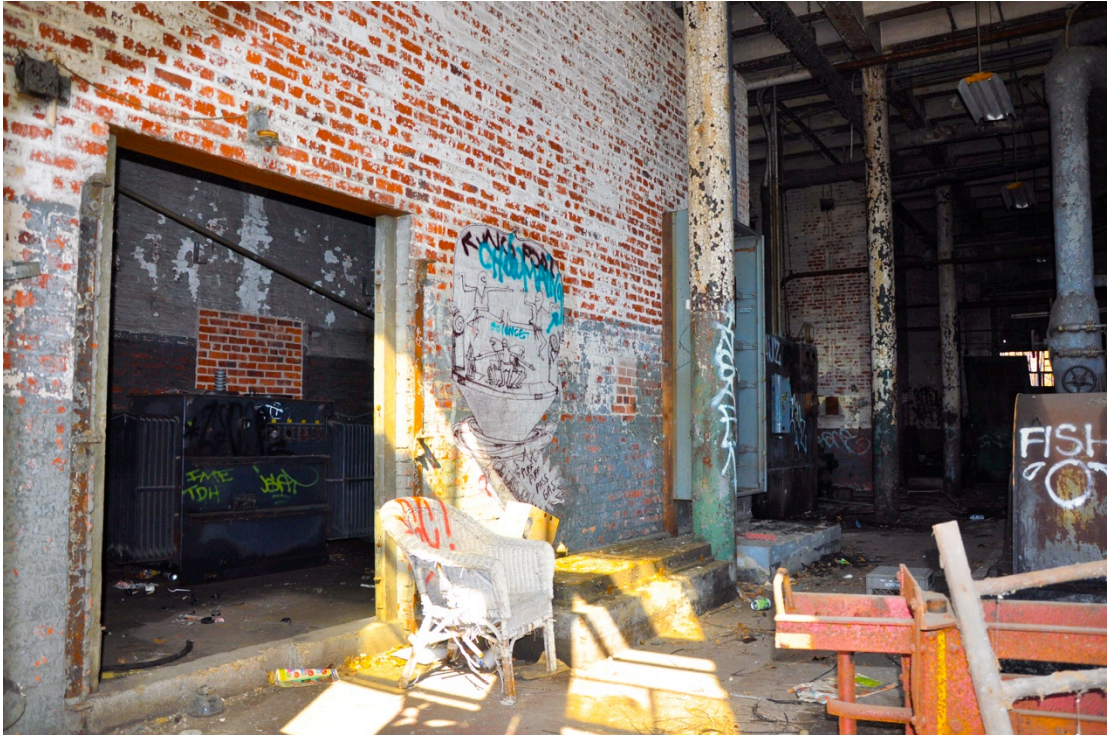
Figure 47: Interior brick walls and graffiti, taken by author
