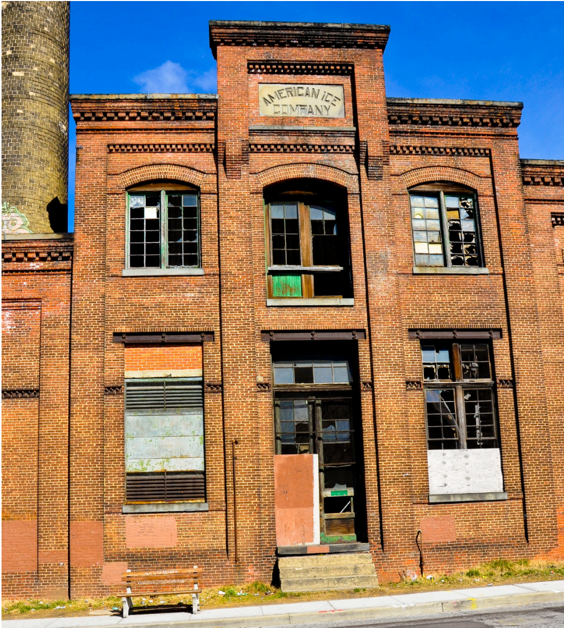
Figure 36: Detail of entrance bay (photo by author).
