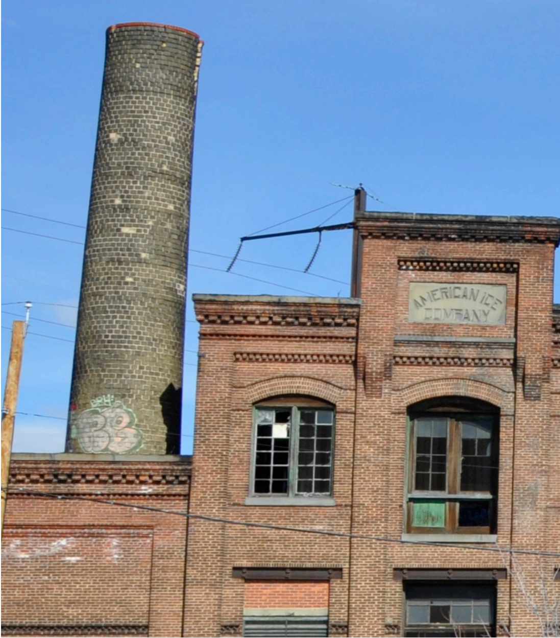
Figure 32: Detail of truncated smokestack (photo by author).
