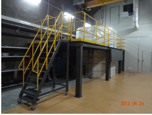
(a) The passive shielding with platform
