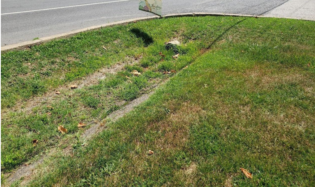
Figure 5.16 “Existing Concrete Swale along Deale Churchton Road”
