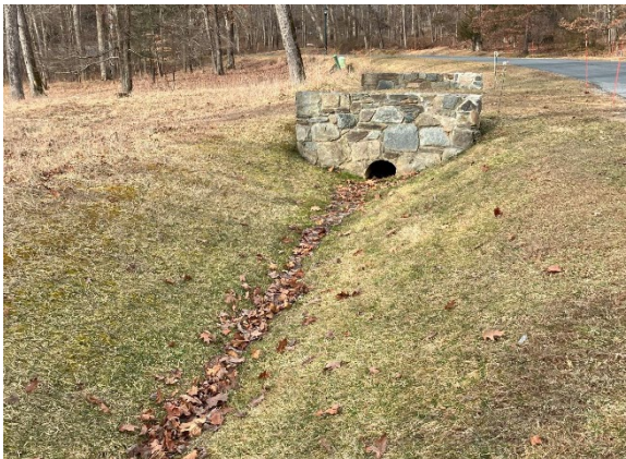
Figure 2.24 Stormwater channel with bridge from previous residential driveway
