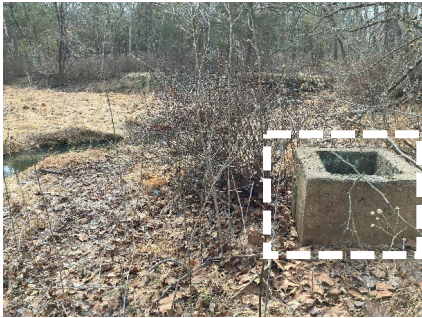
Possibly old pond overflow system
