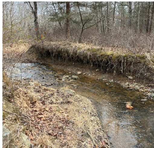
Figure 2.28: Heavily eroded bank where Greenbriar Branch exits the pond basin. Bank cliff is approximately five feet tall.
