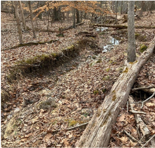
Figure 2.27: Intermittent creak showing signs of erosion
