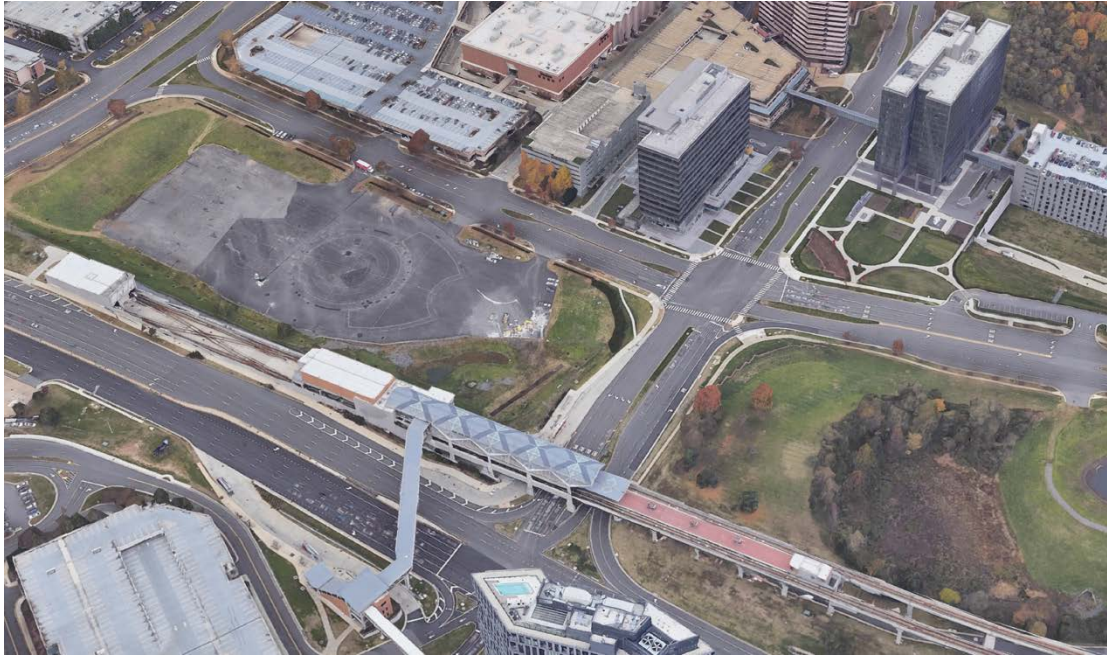
Fig 87. Lerner Square at Tysons II – Before (Source: Jefferson Choi)
