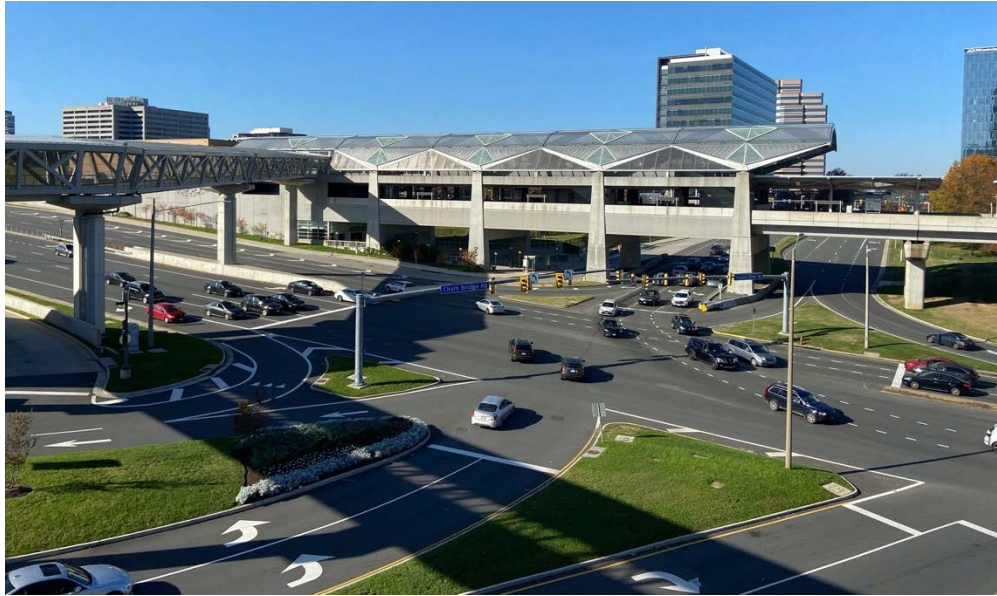
Fig 18. Tysons Metro Station (Source: Jefferson Choi)
