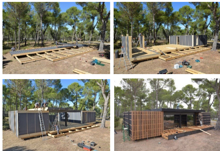
Figure 12: Series showing Pop-Up House construction (Multipod Studio)
