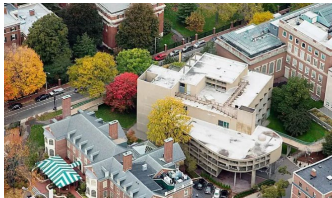
Figure 3: Carpenter Center for Visual Arts (Credit: ArchDaily)
