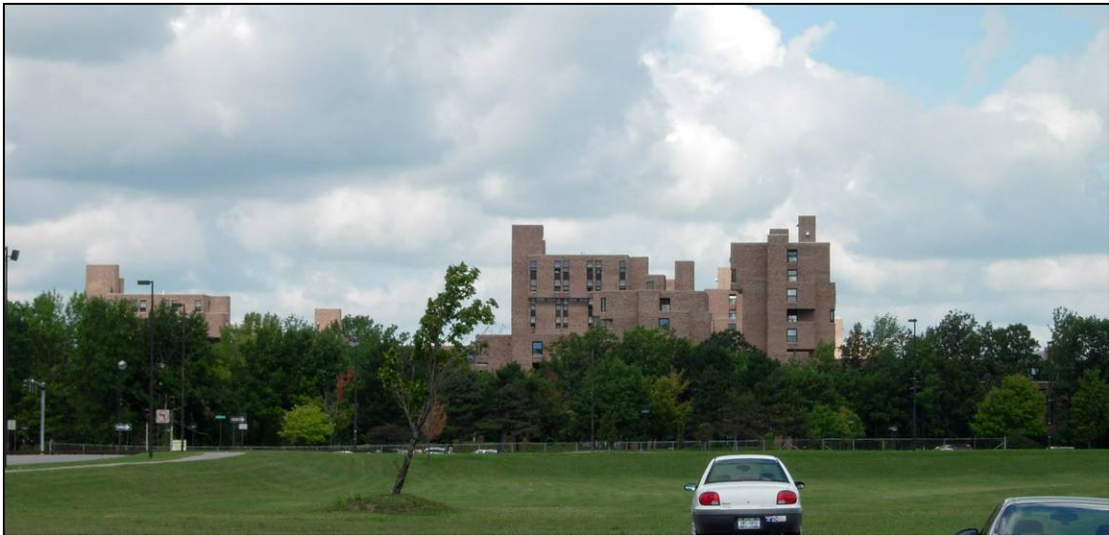
Figure 46: View looking north at Ellicott Dormitory
