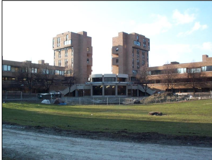
Figure 2: View looking northwest at Ellicott Dormitory.
