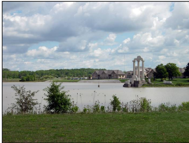
Figure 43: View of Lake LaSalle looking at Baird Point.
