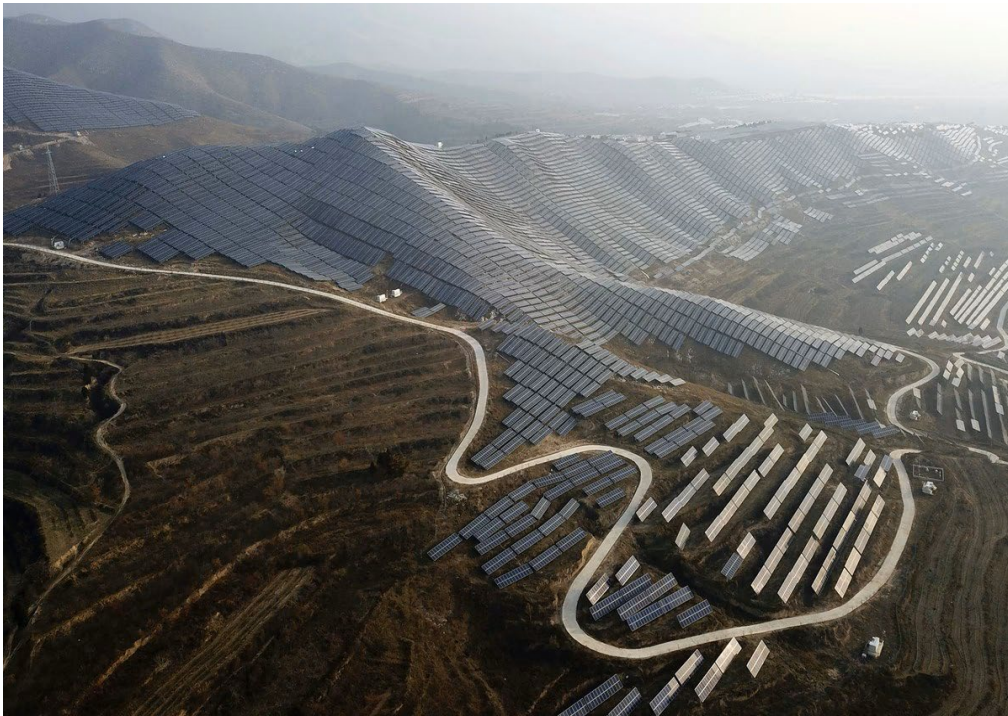
Figure 5. Solar photovoltaic installation in Ruicheng County, Shanxi Province, China (McNeil, 2019)
