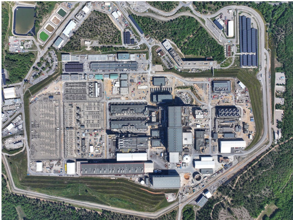
Figure 36. 445-acre ITER campus, in Saint-Paul-lès-Durance, France, aerial image (ITER, 2025)
