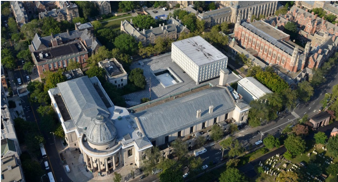
Figure 31. Beinecke Library at Yale by SOM, aerial image (Google Earth, 2025)
