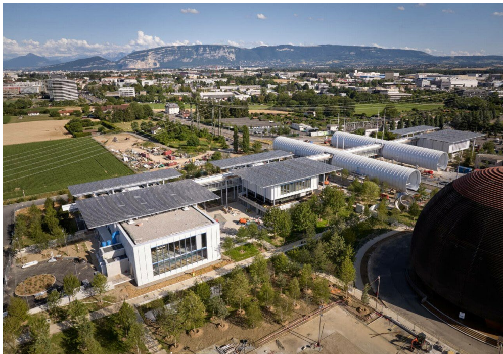
Figure 23. CERN Science Gateway aerial image (RBPW, 2024)
