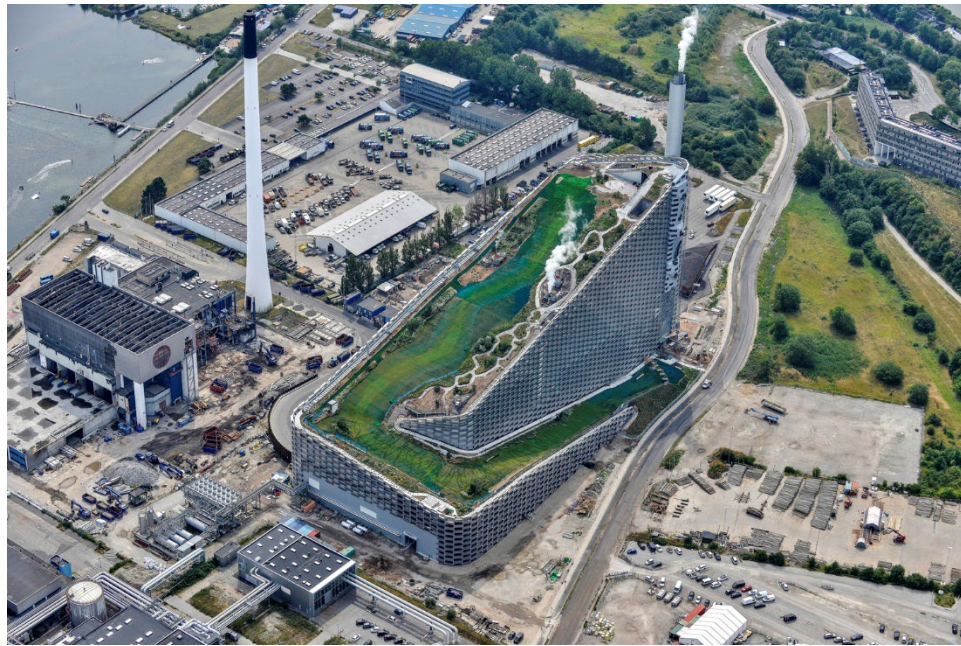
Figure 25. Aerial image of CopenHill by BIG (Google Earth, 2025)
