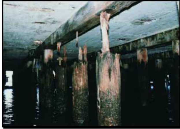
Figure 15: Marine borers (Limnoria) attacking untreated timber piles (FHWA, 2006)
