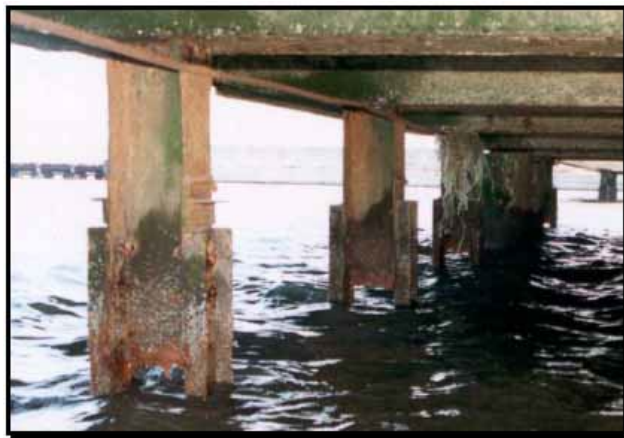
Figure 15: Marine borers (Limnoria) attacking untreated timber piles (FHWA, 2006)
