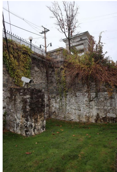
Figure 17. View north of the retaining wall showing different periods of construction. Emory Lane Studio, November 2023.
