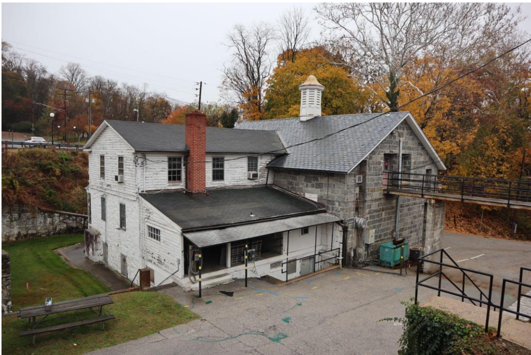
Figure 13. View east showing northwest and southwest facades. Original 1851 jail shown under framed Third floor at the left. 1878 additions in stone building to the right and framed third-floor portion with white siding beyond the chimney. Emory Lane Studio, November 2023.
