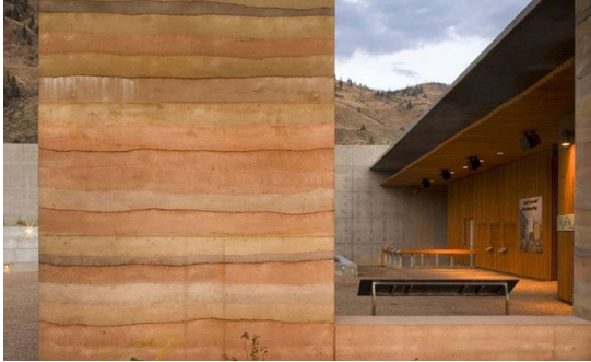
FIGURE 18: Rammed Earth Construction, Nk'Mip Desert Cultural Centre (Source: materialdistrict.com )
