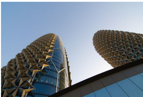
FIGURE 9: Kinetic Façade on the Al Bahar Towers (Source: architecture.org)
