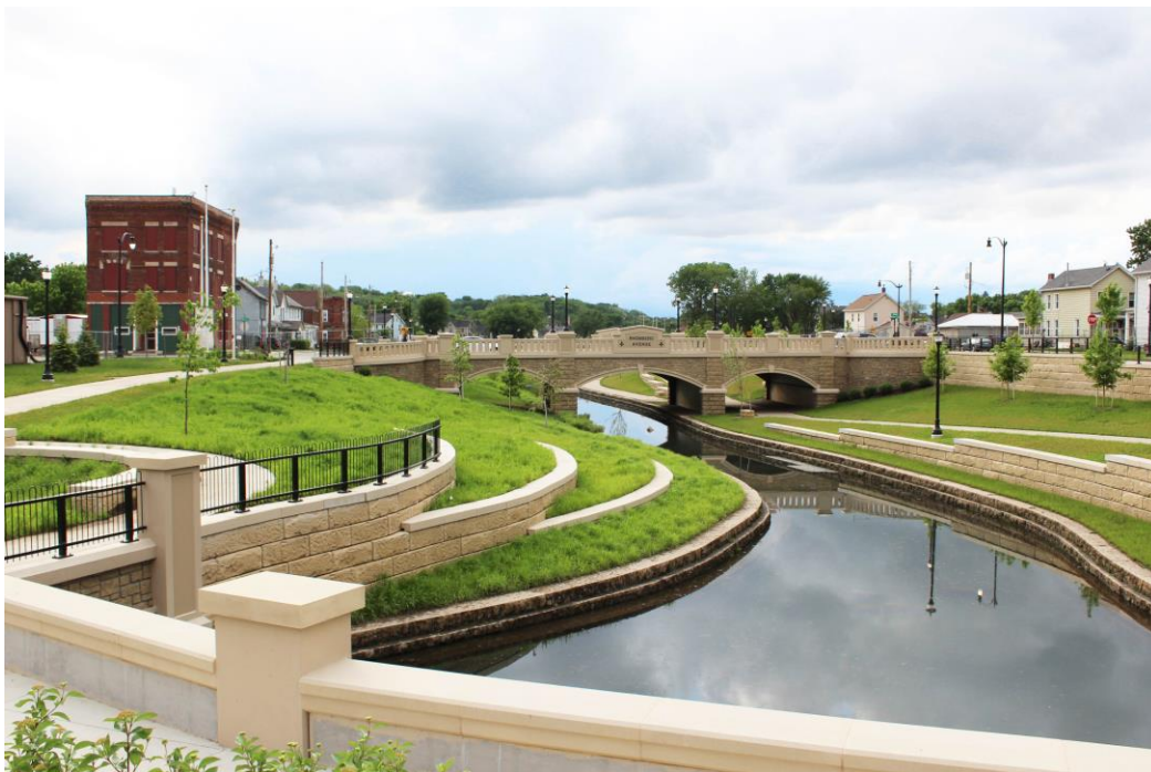
Figure 4.2: Greenway in Dubuque, Iowa - in response to a history of flooding, Dubuque, Iowa, installed the Bee Branch Creek Greenway to control flooding and provide recreational space. (Source:Fourth National Climate Assessment, Photo credit: City of Dubuque, Iowa)
