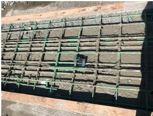
(a) Strain sensors' installation
