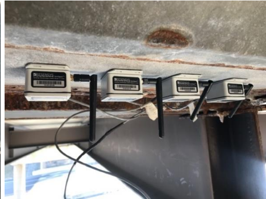
(a) Strain sensors' installation
