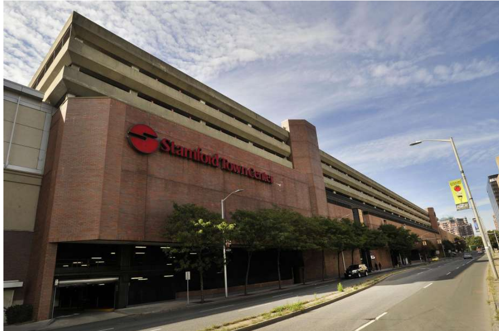
Figure 3: The Stamford Town Center parking garage. The garage spans the entire length of the city block, providing an ample amount of parking, and shielding the mall from the downtown “urban blight” (Source: Jason Rearick via The Stamford Advocate)
