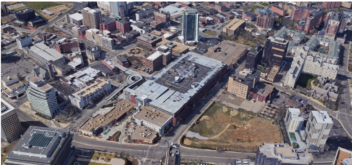
Figure 14: Stamford Town Center Aerial (Source: Google Earth)
