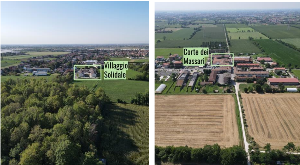
Figure 6: Context photos of the co-housing communities in Lurano and Castel Cerreto surrounded by agricultural land. Source: photographed by author
