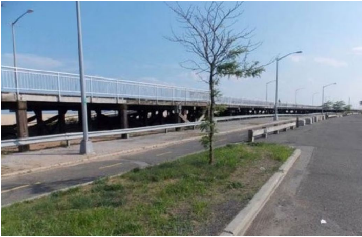
Figure 6.9. Image of Existing Boardwalk Conditions (USACE, 2022)
