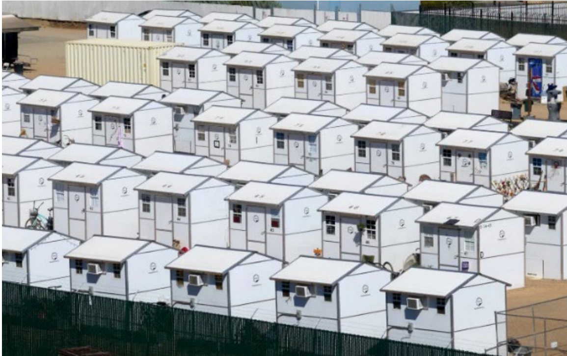
Fig. 1.3 – Tiny homes that are prefabricated modular housing systems in California Greaves, Fred. 2023. CBS8.
