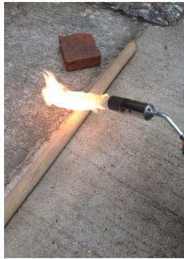
1. Fire stripped bamboo to become malleable without burning the bamboo piece
