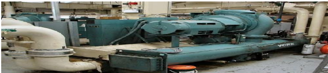
Figure 5.4 - Typical York Chiller Installed in the 1970's
