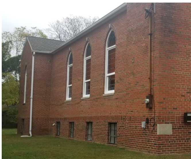
Figure 13: West Elevation/Facade, (View from parking Lot) Photo Credit: Author
