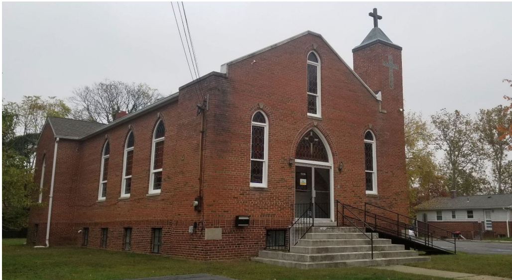
Figure 14: First Baptist Church in its surrounding landscape Photo Credit: Author
