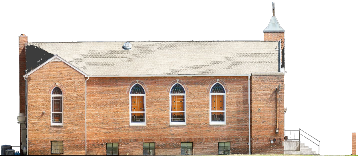
Figure 32: Orthographic projection/Wast elevation of First Baptist Church Source: Author
