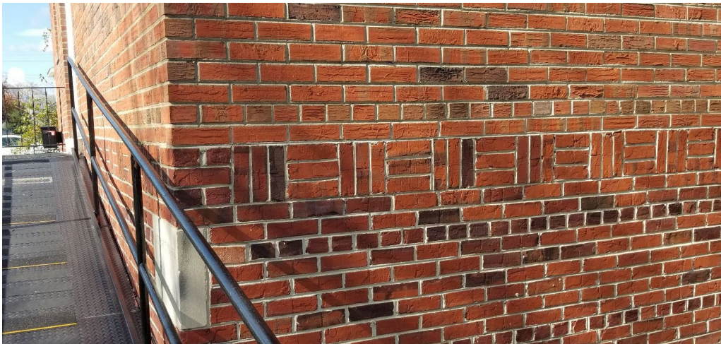
Figure 7: Basketweave, brick bond indicating a change in level. Photo Credit: Author
