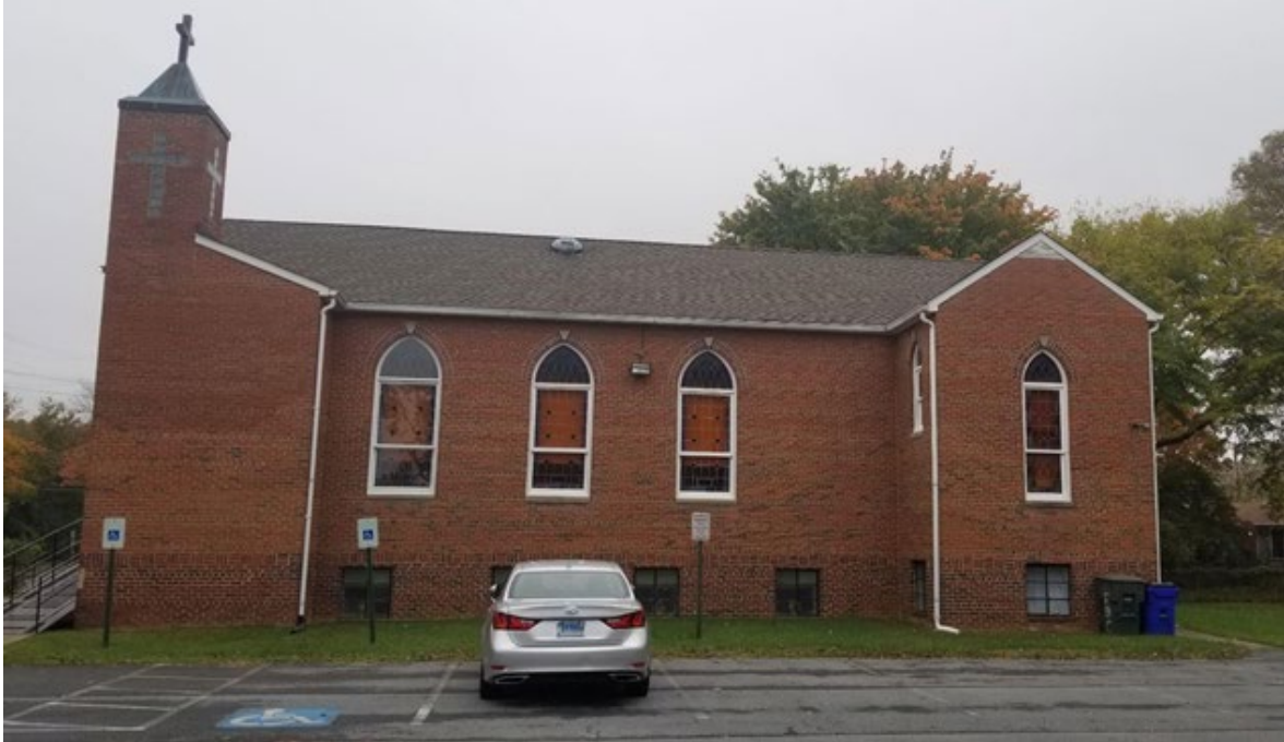
Figure 11: East Elevation/Facade, (View from parking Lot) Photo Credit: Author
