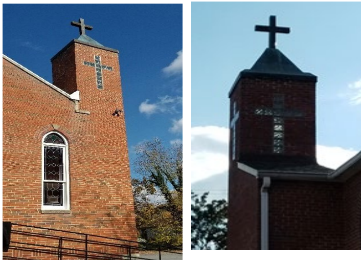
Figure 10: Brick Steeple, with Aluminum capping. Photo Credit: Author
