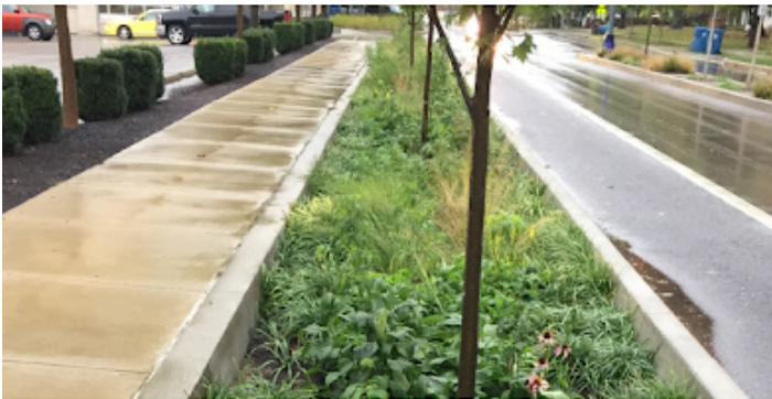
Figure 137: Photo of Sunken Bioretention Along Urban Street
