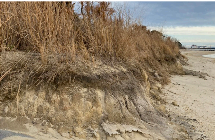
Figure 7: Shoreline Erosion Along Point Lookout
