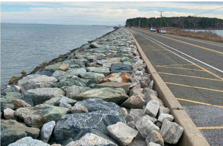
Figure 12: Bulkheads at Point Lookout
