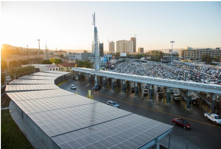
Figure 5.8 San Ysidro Land Port roof covered by PV panels
