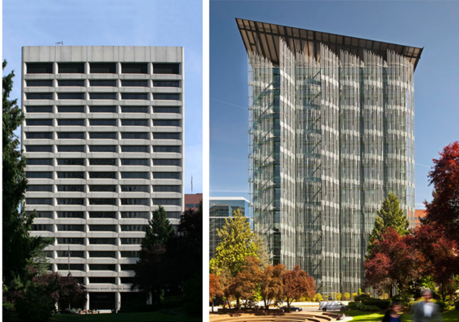
Figure 7.3 building envelope renovation before (left image) and after (right image)
