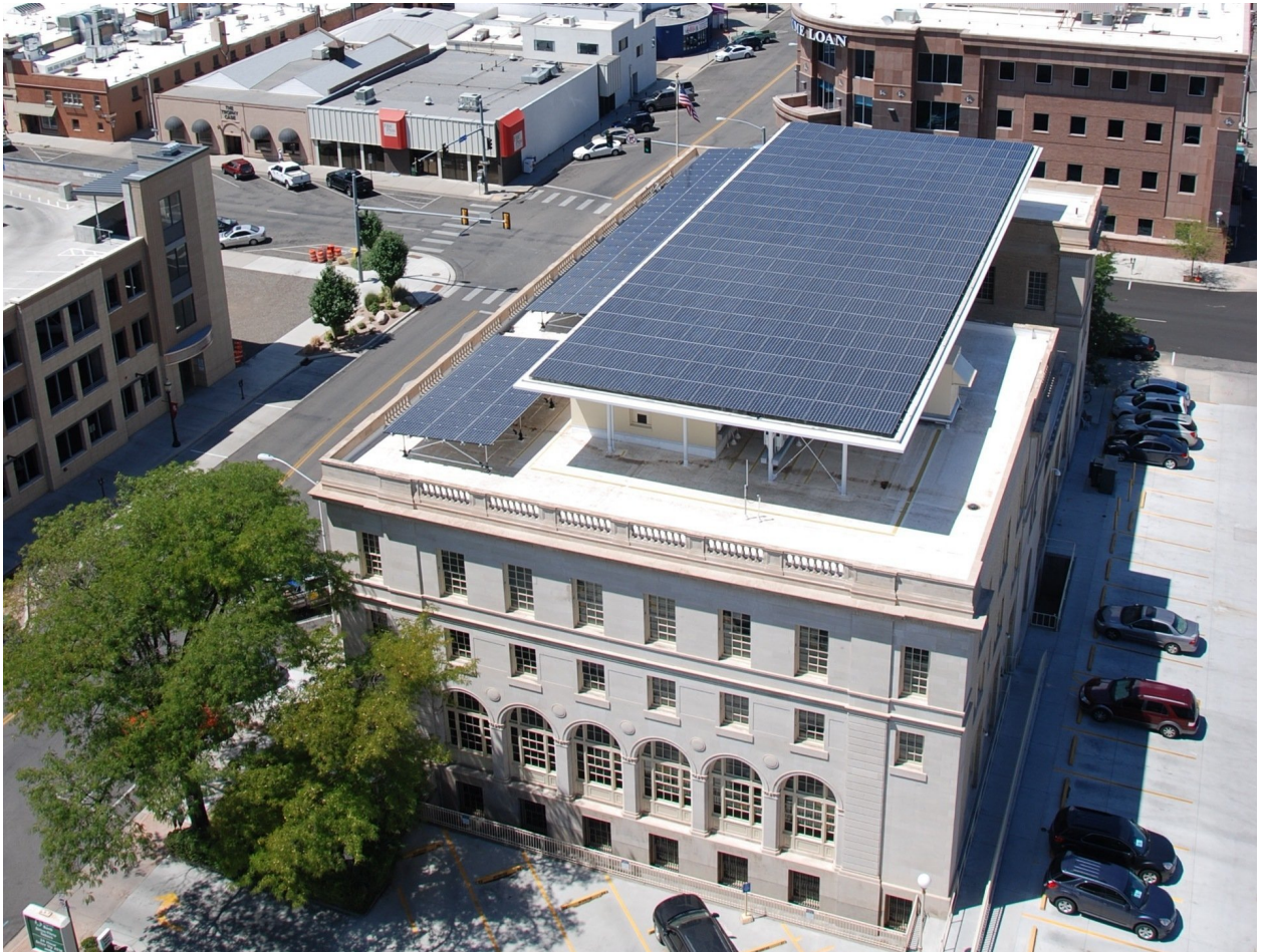
Figure 7.1 Roof mounted solar panel
