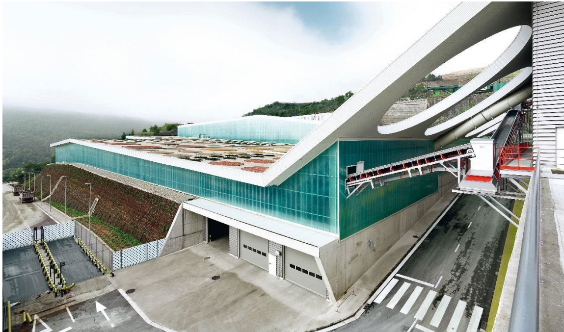
Figure 10: Waste Treatment Facility
