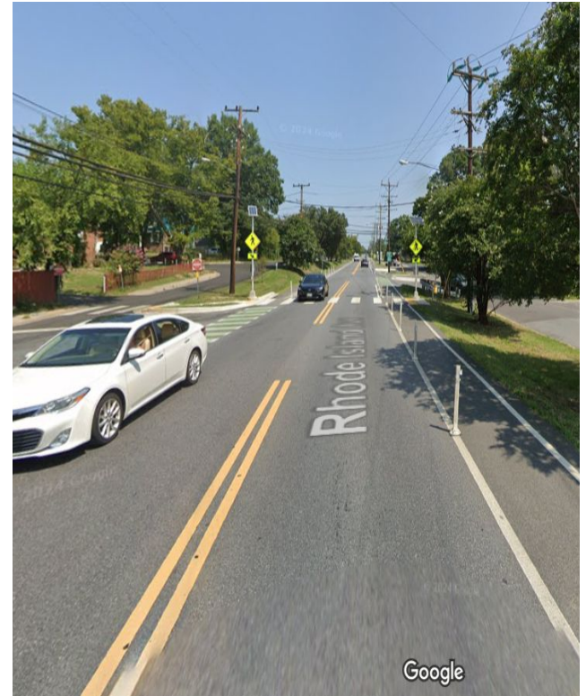
Recently Constructed Bike Lanes on Rhode Island Avenue, College Park, MD
