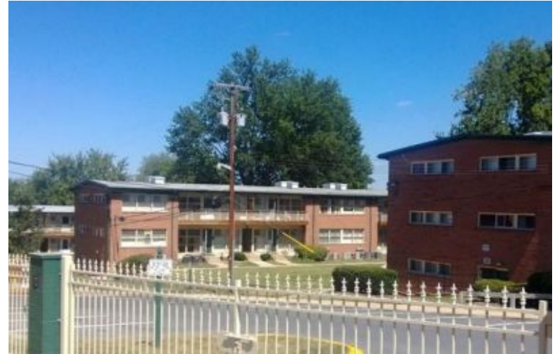
University Gardens Apartments, one of 13 apartment complexes in Langley Park. Source: CASA
