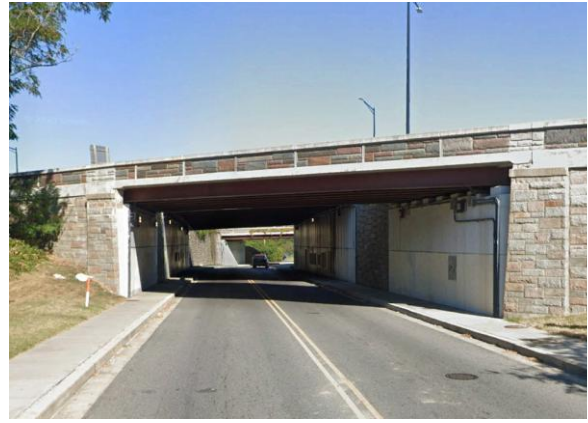
Figure 80: Nicholson St. Underpass. Credit: Google Earth.
