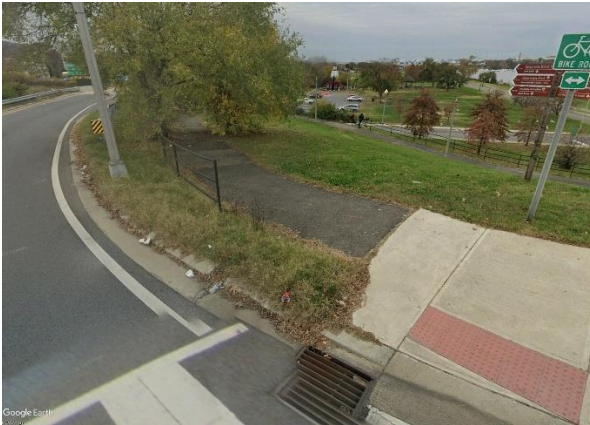
Figure 82: Entrance to the Park looking from the John Phillip Sousa Bridge. Credit: Google Earth.
