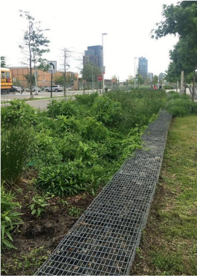
Figure 20: Rock-filled gabions are set in a planted swale along Central Boulevard to interrupt and slow large volumes of rain and storm surge from the neighborhood, as well as filter sediment before it drains. Credit: DuRussel (2018).
