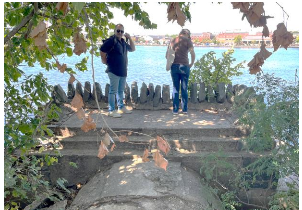
Figure 104: Overlook Area Over Storm Sewer. Credit: the author.
