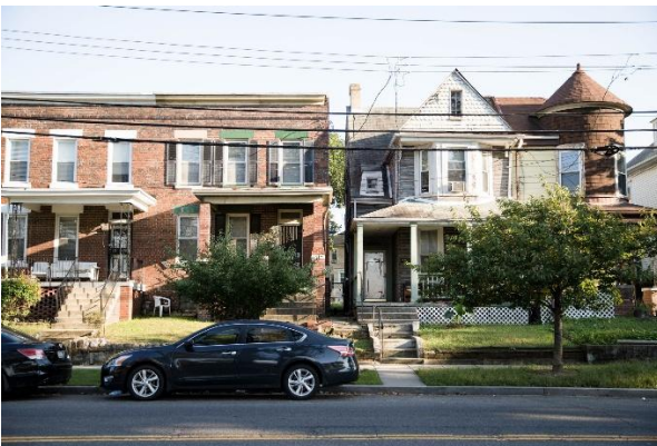
Figure 56: Mix of architectural styles in Fairlawn homes.
