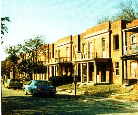
Fig. 150 – Before Redevelopment (Zelinka and Brennan)
