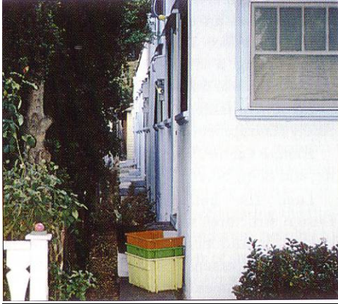
Fig. 7 – Poor design allows undetected access to residential units (Zelinka and Brennan, 2001)
