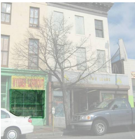
Fig. 84 – Bars on storefronts
