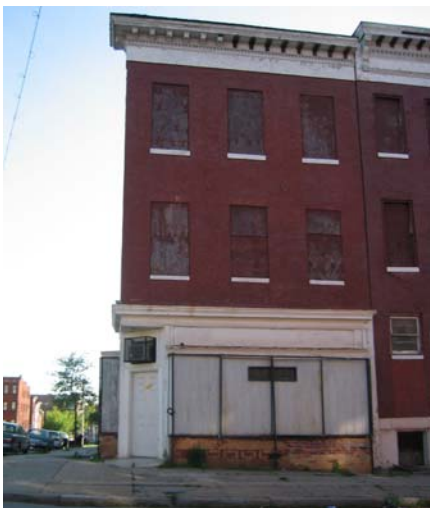
Fig. 254 – Existing vacant corner store
