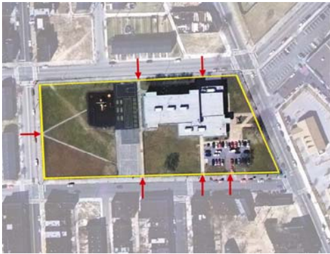
Fig. 131 – Entry points through fence
