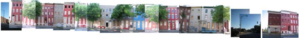
Fig. 107 – Southwestern edge of residential block.
