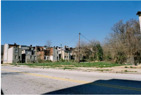
Fig. 112 – Rear of Housing Units
