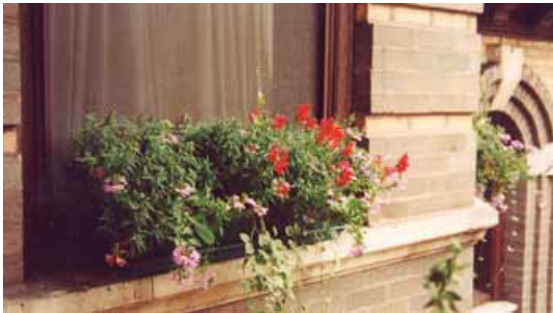
Fig. 235 – Window Box adds life to the unit
