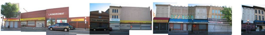
Fig. 78 – Existing buildings along the northeastern side of Pennsylvania Avenue
