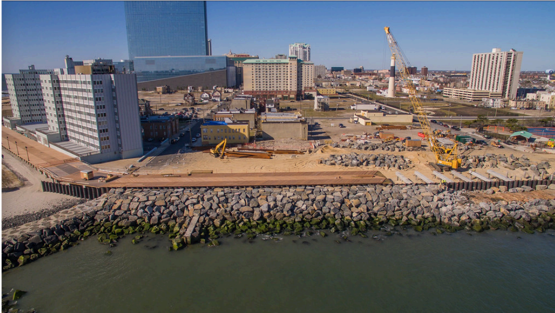
Fig. 3, Atlantic City's North Inlet neighborhood, construction of 1,340 foot seawall and Boardwalk after Superstorm Sandy damage, 2017 (Source: U.S. Army Corps of Engineers)
