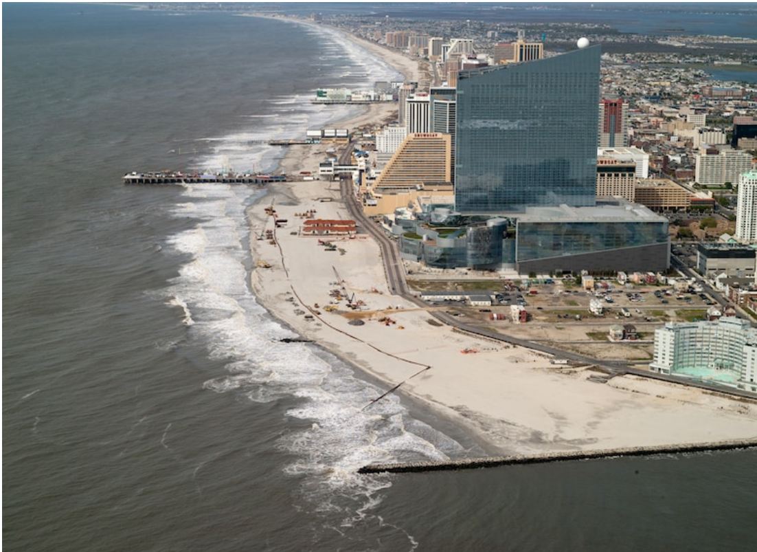
Fig. 4, Jetty (bottom of photo) protects the inlet channel and acts as a deposition catchment, 2018 (Source: USACE)
