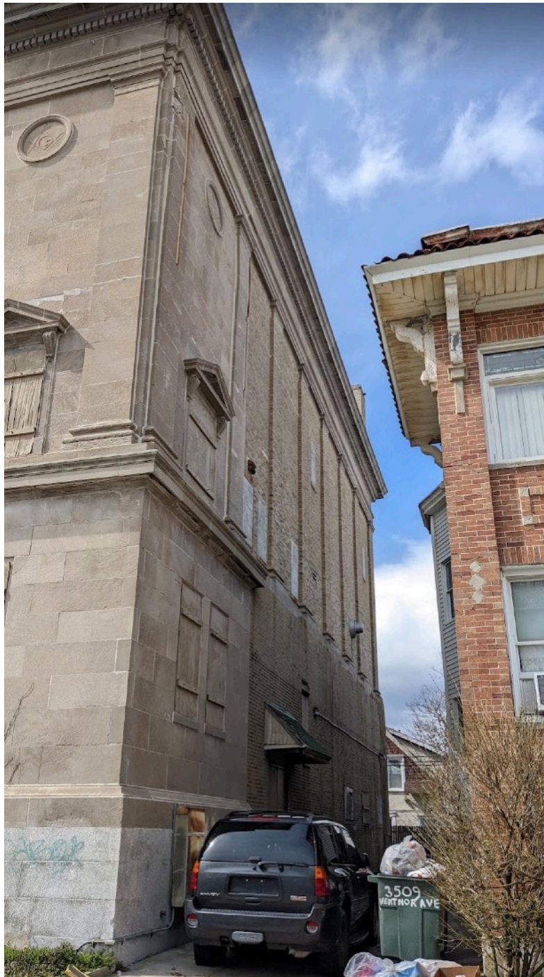
Fig. 23: Front facing photograph of elevation not possible due to neighboring property, March 2022 (Source: Author)
