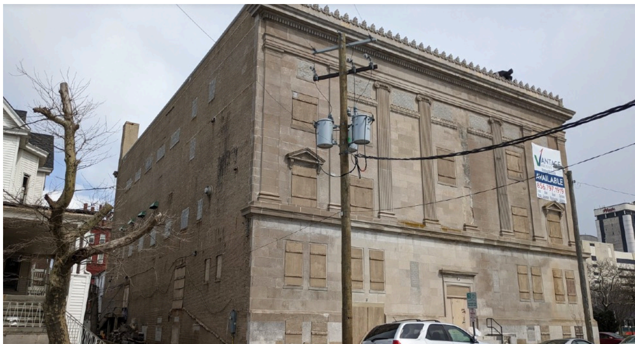
Fig. 19: The northwest corner reveals the change in facade material and ornamentation. The rear (north elevation) faces an alleyway and most utility openings have been cut into this elevation, March 2022 (Source: Author)
