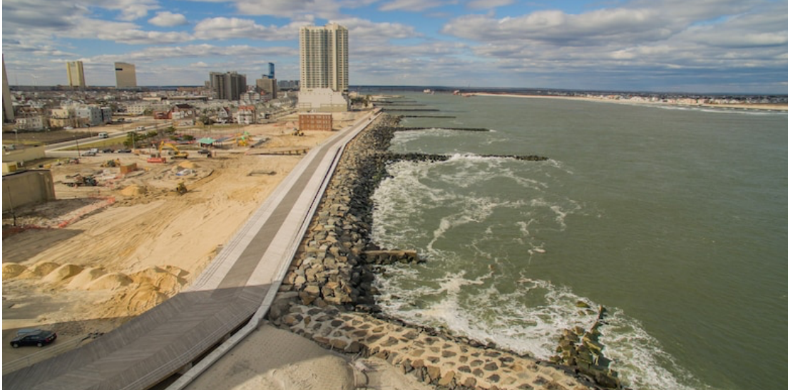
Fig. 2, $40 million seawall and revetment project along Atlantic City's North Inlet, 2018
