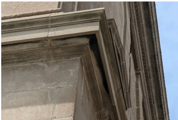
Fig. 12b: Biological growth above and below cornice
