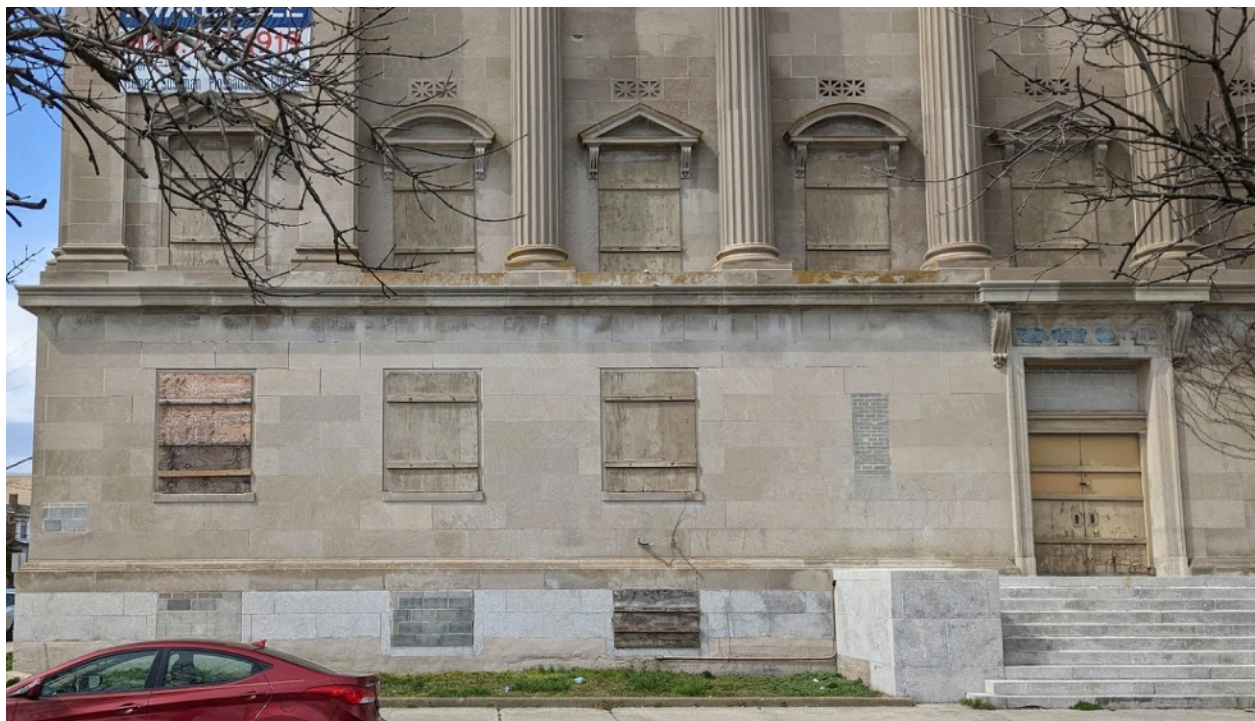
Fig. 6: Granite water table and steps; Indiana limestone upper facade, March 2022 (Source: Author)
