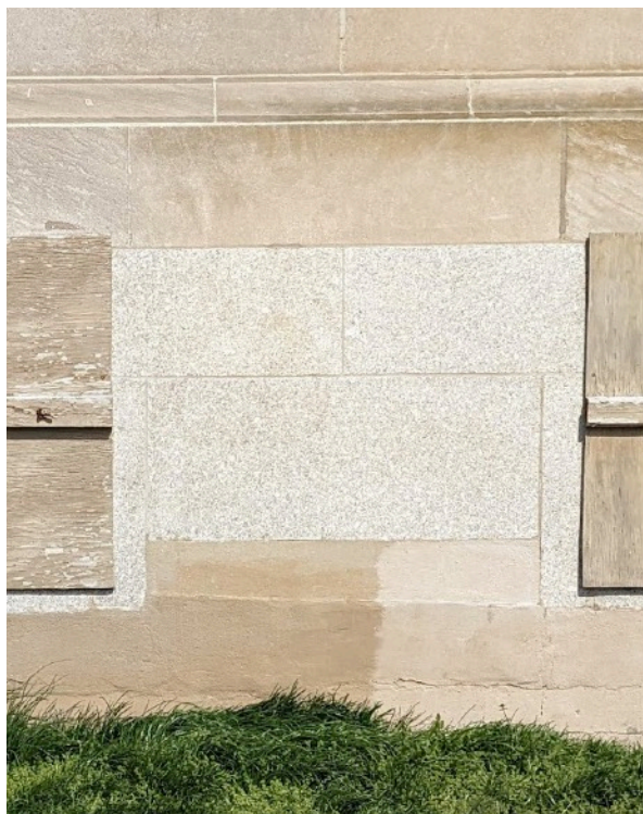
Fig. 16a: Concrete repairs to the granite water table, March 2022 (Source: Author)
