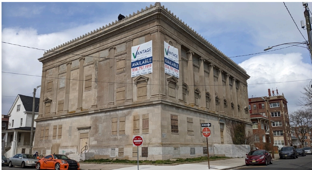
Fig. 14: The public facing front elevation and side elevation provide a continuity at the southwest corner of the Masonic Temple. These are the only two public facing facades and are clad in granite, Indiana limestone, and Ionic ornamentation, March 2022 (Source: Author)
