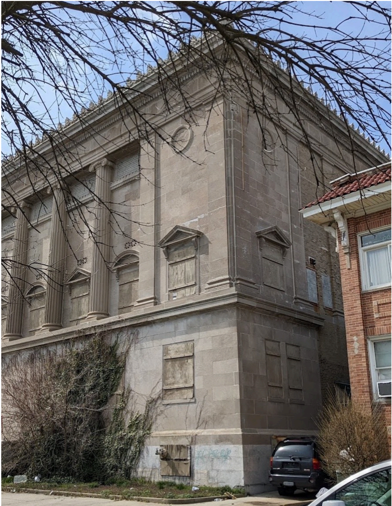
Fig. 25: Alternative view of southeast corner showing transition from limestone front facade to brick faced side facade, March 2022 (Source: Author)
