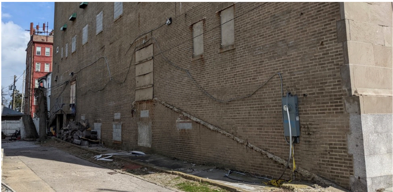
Fig. 8: Tan brick laid in a running bond pattern on the less visible facade, March 2022 (Source: Author)
