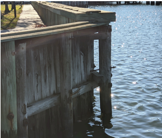
Fig. 3, Left: Wood bulkhead in disrepair, 2021 (Source: Author) Right: New steel sheet pile bulkhead, 2021 (Source: Author)
