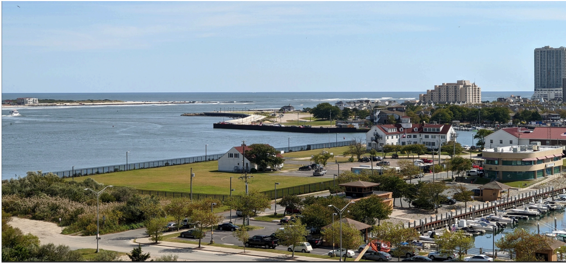
Historic Coast Guard Station, Atlantic City, 2021 (Source: Author)
