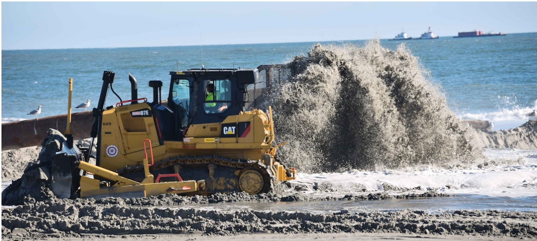
Fig. 5, Beach replenishment in Ocean City NJ, c. 2018 (Source: USACE)
