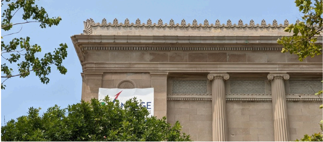
Fig. 7: Detail of Indiana limestone at entablature and parapet, July 2021 (Source: Author)
