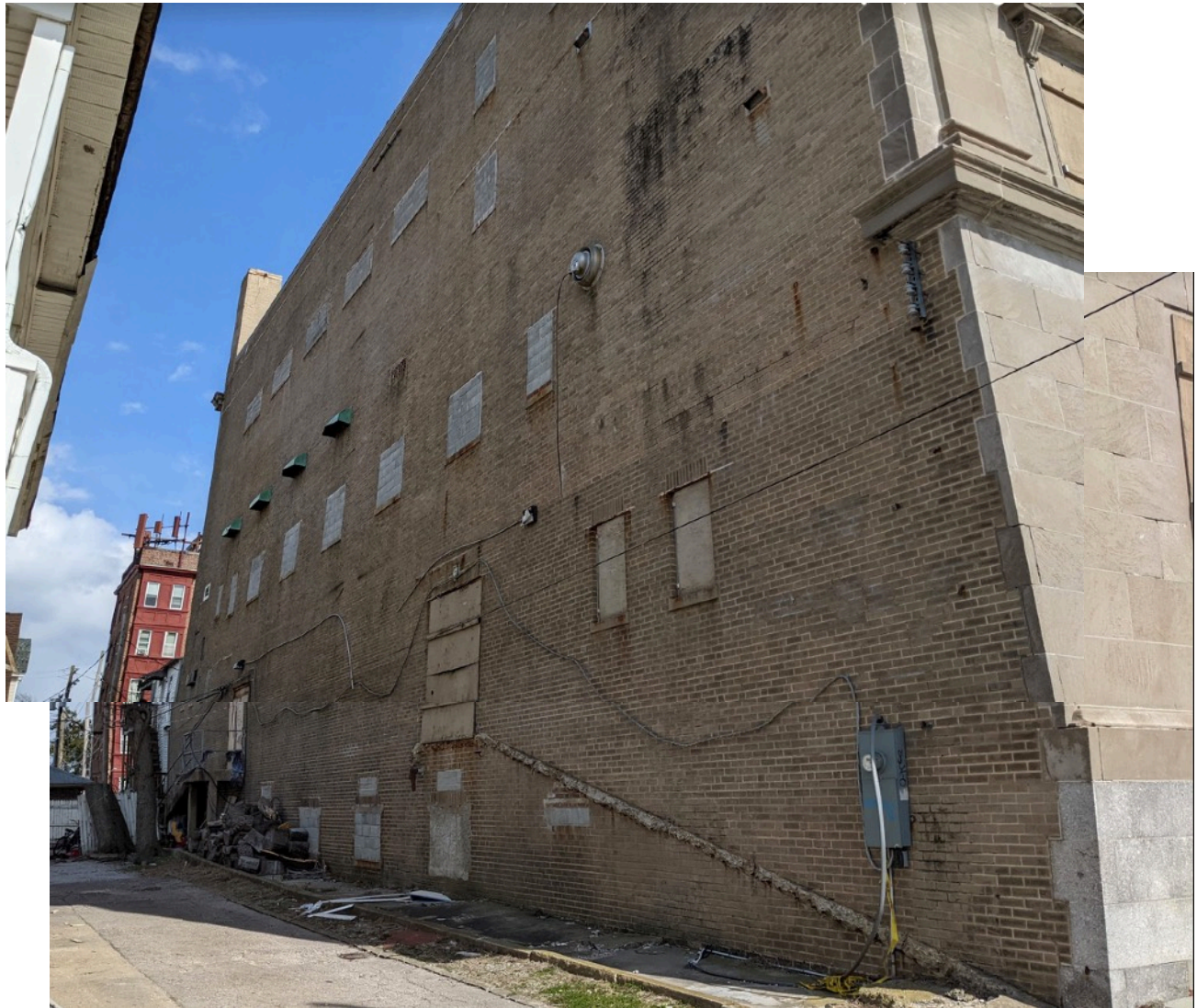
Fig. 20: Rear elevation, March 2022 (Source: Author)
