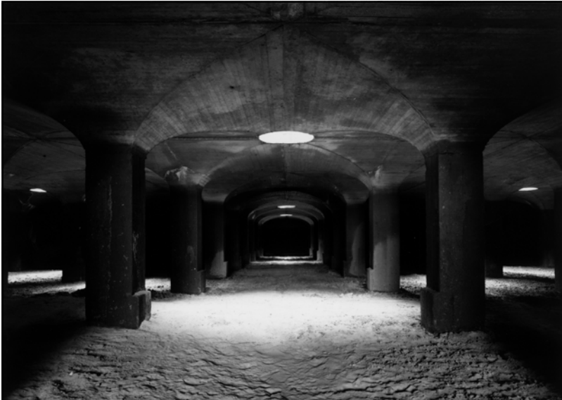
Interior of typical underground water filter cell (photo: Anice Hoachlander, copyright 1990)
