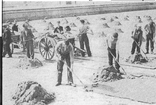
Removal of schmutzdecke, Collins, p87
