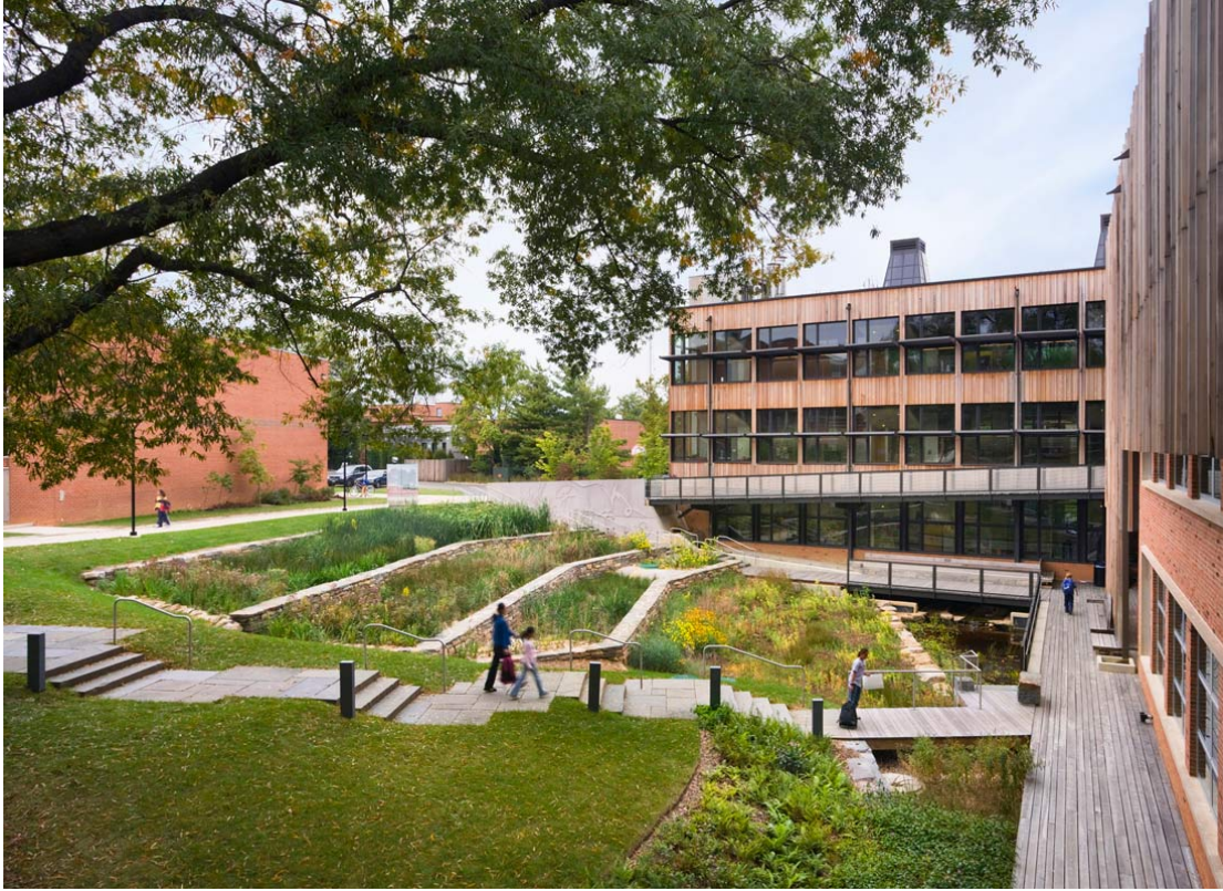
Figure 27: A constructed wetland at Sidwell Friends School treats building wastewater and recycles it for grey water use within the building (Image credit: Albert Vecerka/Esto)
