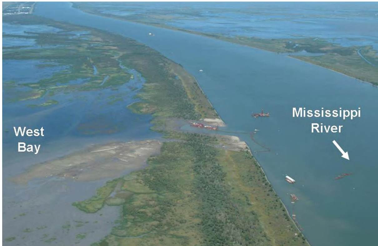
Figure 3 : Image of the West Bay Sediment Diversion. (Source: USACE)
