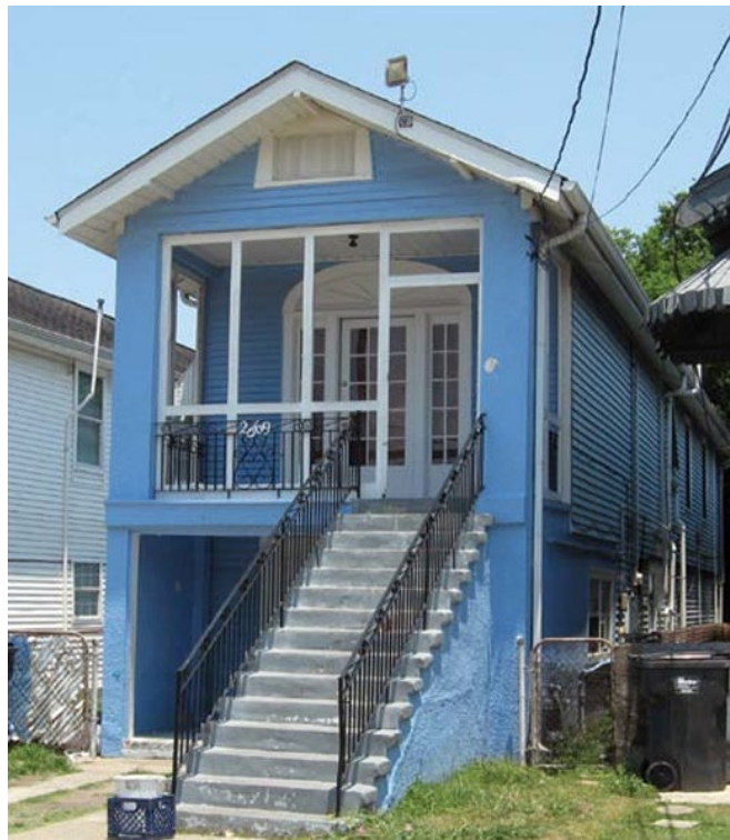
Figure 12: Raised basement shotgun house (Source: FEMA)
