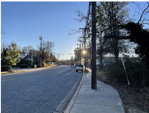
Figure 35. Typical Condition of No Buffers Between Vehicular and Pedestrian Lanes. Source: Ada, 2023
