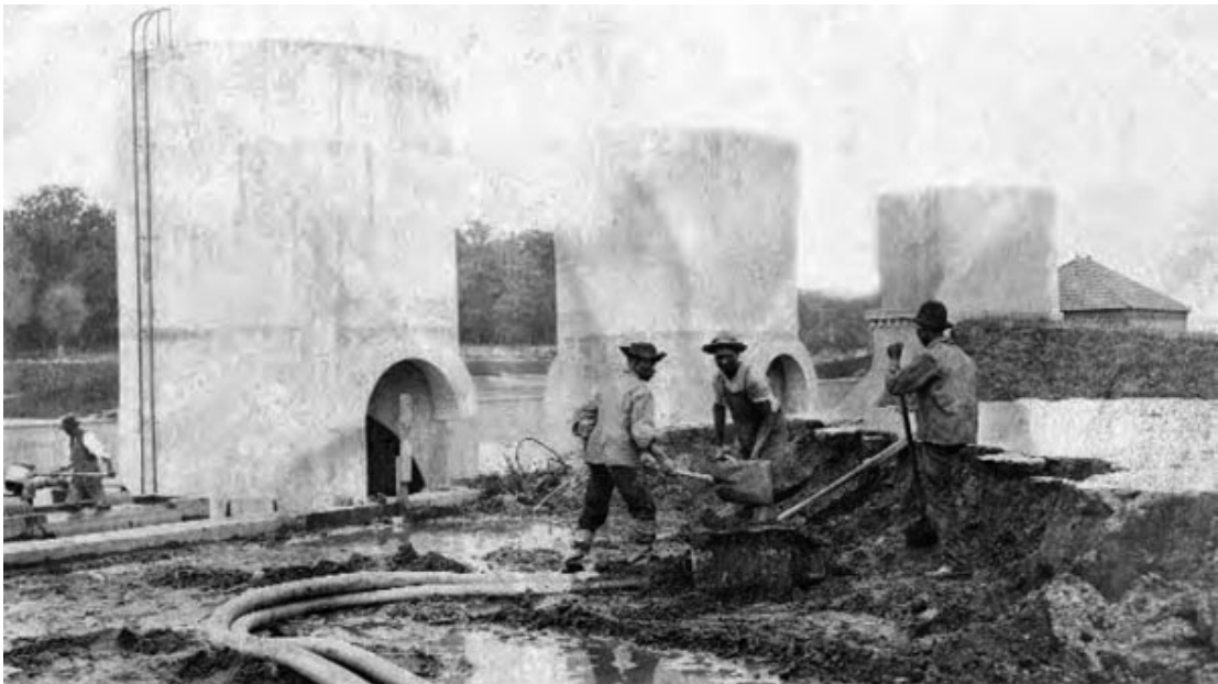
Figure 33: Workers constructing sand filtration towers at McMillan Reservoir Image courtesy of friendsofmcmillan.org .
