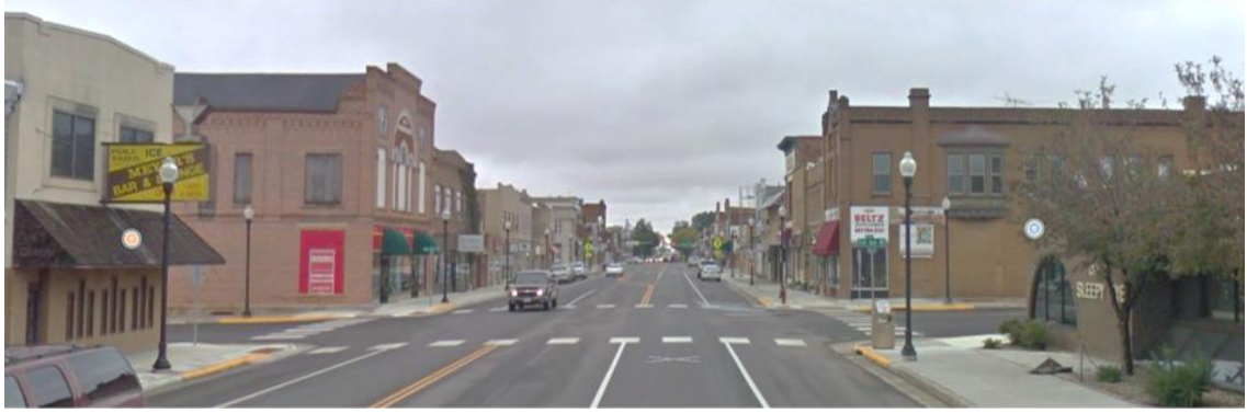
Figure 3.33. Existing eastern end of Main Street looking West
