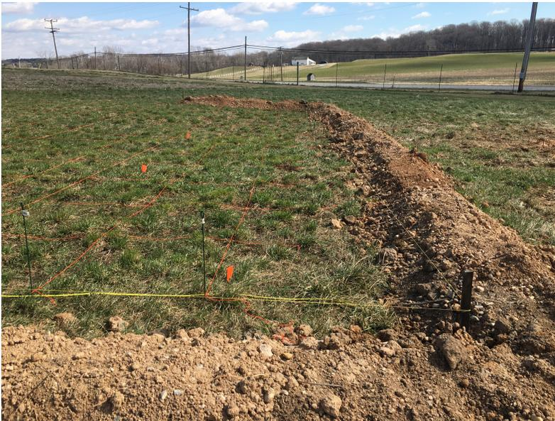
Figure 4.3 Example of soil berm built to contain floodwater.
