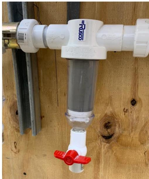
**Figure 3B:** Rusco Spin-Down Filters (74 microns).
