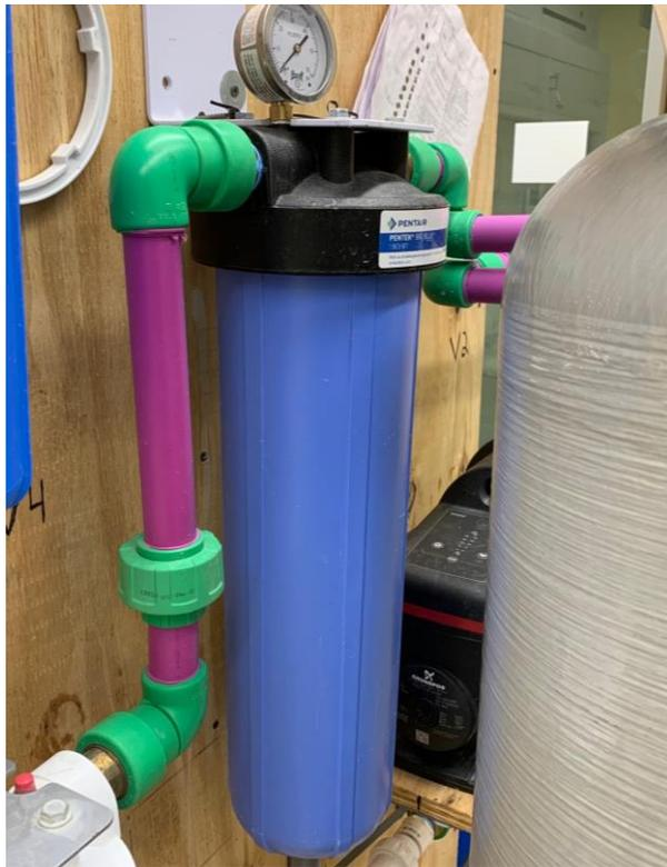
**Figure 3E:** One Micron Bag Filter.
