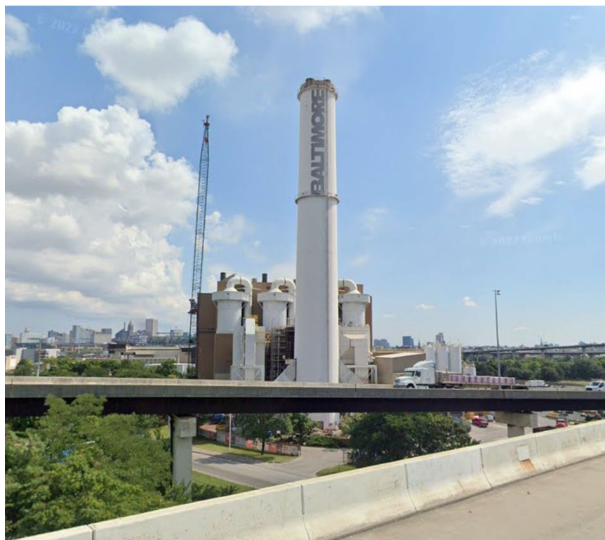
Figure 15: View of Wheelabrator Incinerator from I-95 (Google Maps Street View)
