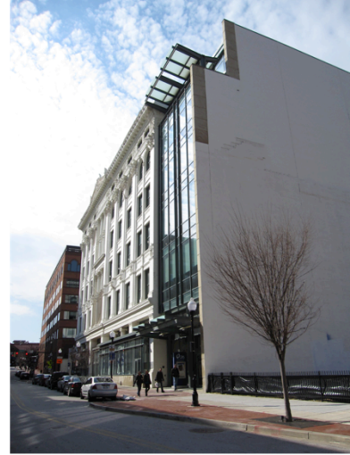
View of adjacent building to the west
