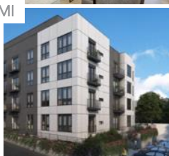
Villages - Morgan Blvd Stations
