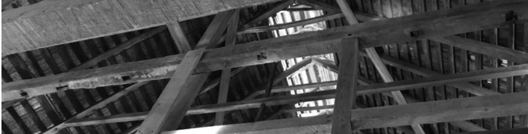
Figure 4. Cremona Barn 1, Ghost Mortises for Studs and Door Posts on East Girt.
