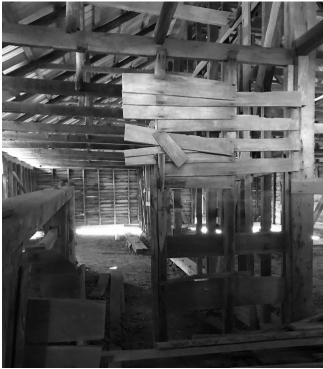
Figure 18. Plumer-Cranford Barn, View of Riven Clapboard Siding on Partition Between East and South Sheds.
