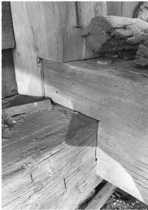
Figure 31. Trott Barn D, Southwest Door Post, showing intermediate sill lapped and tenoned into side wall sill.
