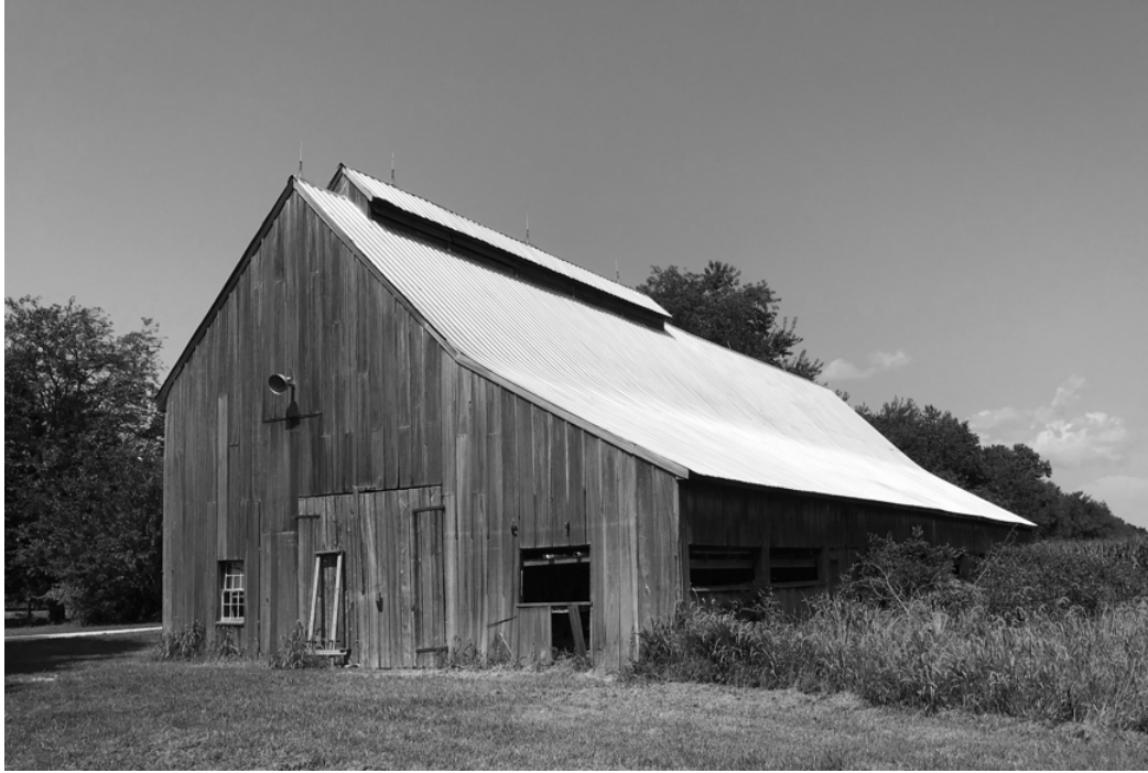
Figure 2. Cremona Barn 1, Southwest Elevation; the original portion of the barn is one-half of the gable-roofed section on the left.
