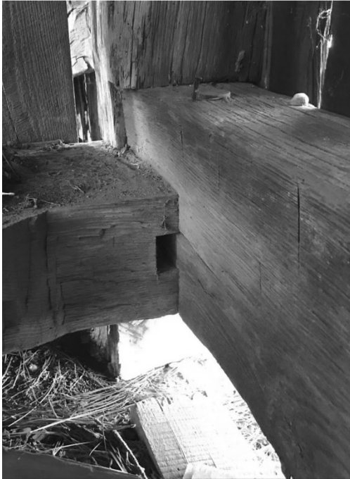
Figure 30. Buckler Barn, Southwest Corner Post, showing the mortise in the side wall sill, with a peg through the end sill, and the lapped corner post.
