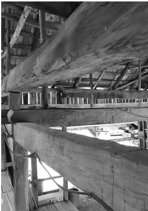
Figure 20. Half Pone Barn, Double Joist Framing Over Eastern Intermediate Sill Posts.
