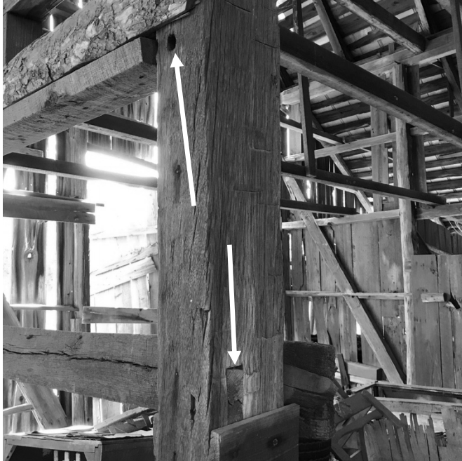
Figure 15. Buckler Barn, Used Pintle on North Wall Door Post and Mortise for Siding with Remnant of Tenon.
