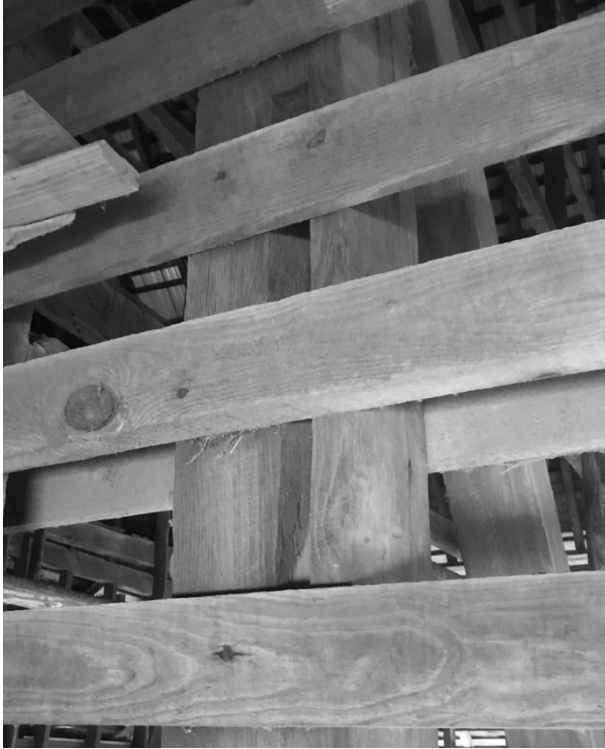
Figure 8. Cremona Barn 2, Tall Mortise for Steep Downbrace into South Shed.
