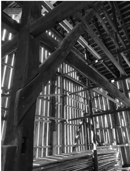
Figure 29. Hallowing Pt. Barn A, Upbrace Connecting to Post.
