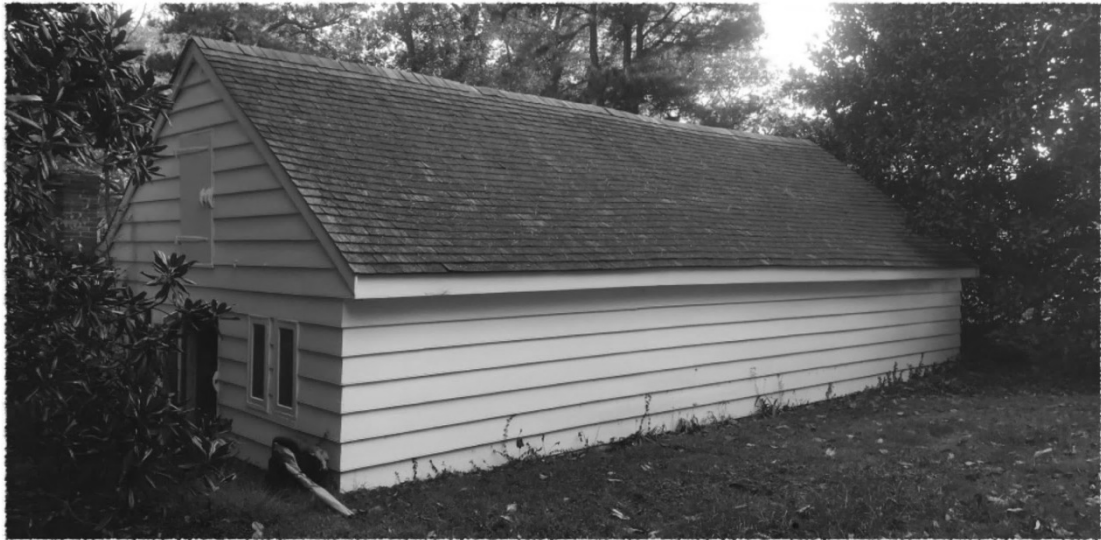
Figure 36. Cremona Livestock Barn, Northeast Elevation; the siding was renewed in the 1930s, and a low shed was added running along the south wall.
