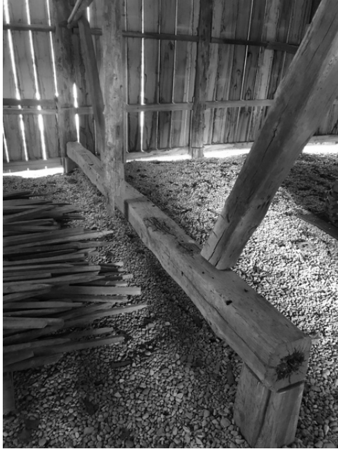
Figure 27. Dawson Barn, Intermediate Sill with Earthfast Posts.
