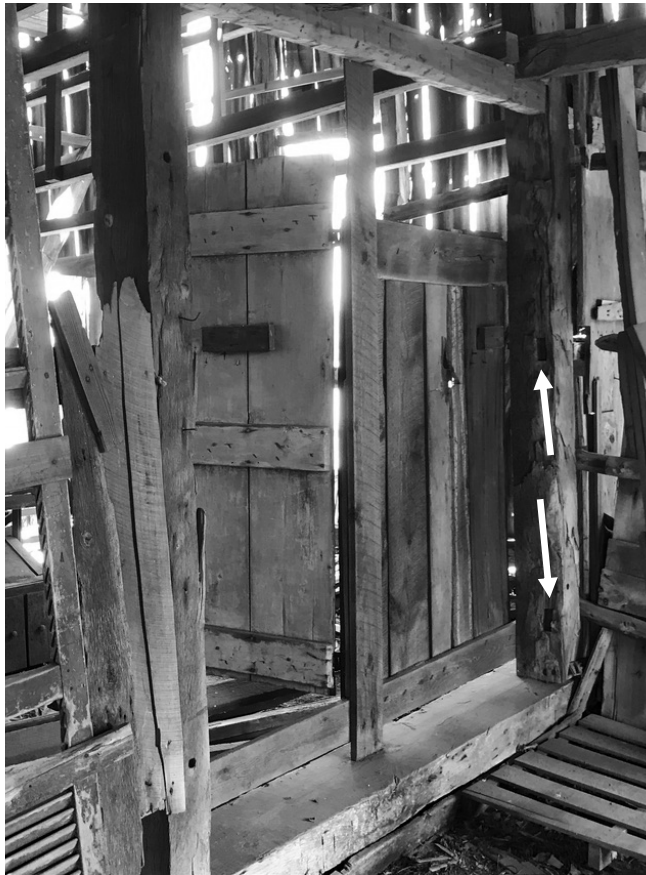
Figure 16. Buckler Barn South Doorframe from Shed Showing Riven Siding and ghost mortises on Door Post for Nailers Across the Doorway.
