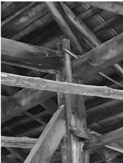
Figure 33. Vieley Barn Clenched Joint at Plate with "Rabbit Ears."
