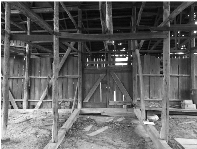
Figure 25. Trott Barn D, Center Aisle facing South and Showing both Intermediate Sills and Double Doors to Shed.
